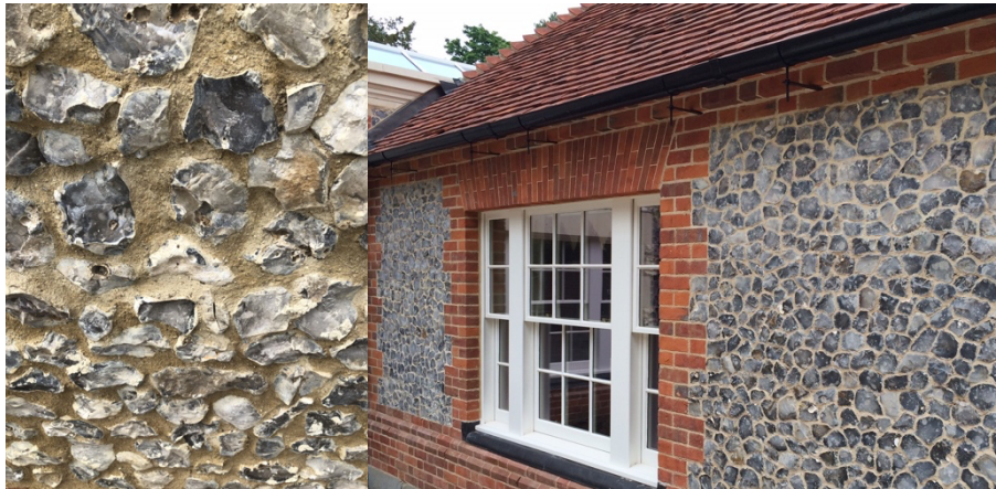
Flint work - mixture of knapped Chalk and Field flint 3-6 inch
