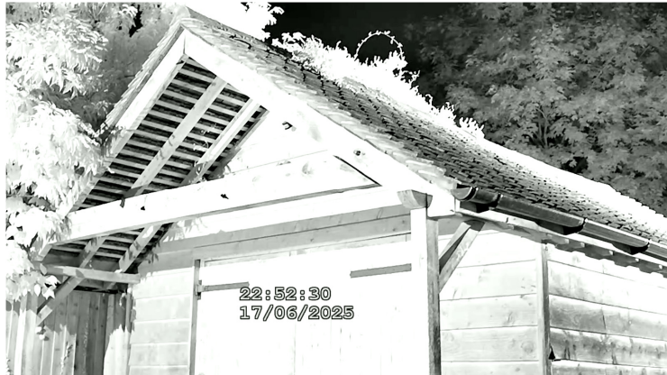
Sionyx Aurora Pro at Surveyor Location 1.
