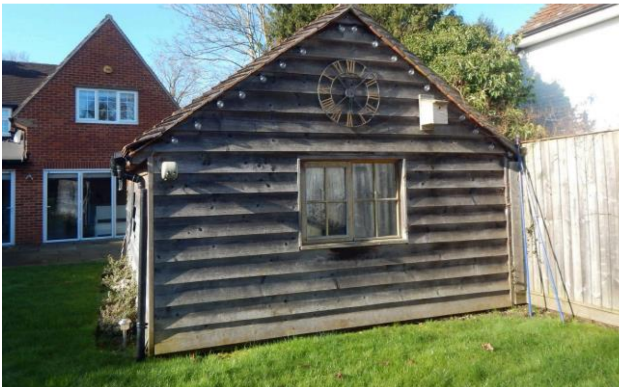
Image 2 – East facing elevation of the structure
