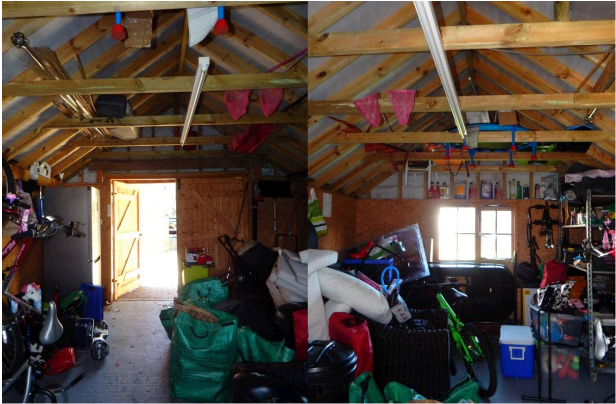
Image 7 – Internal views from within the structure
