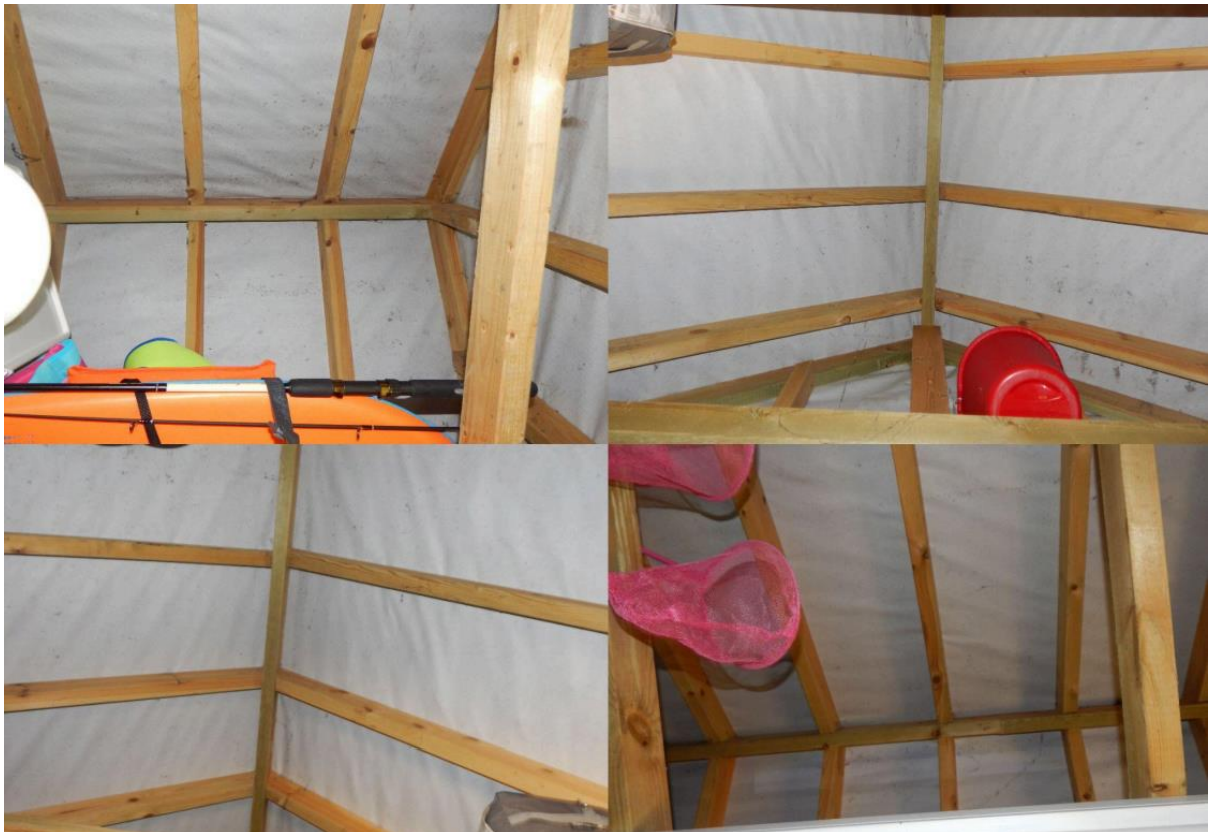
Image 8 – Internal views from within the structure
