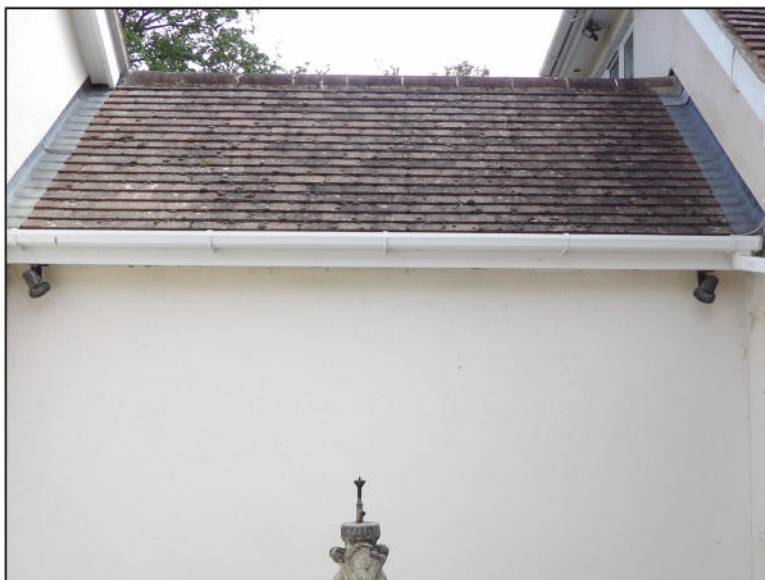
Figure 12. Sealed roof and ridge tiles on connecting building and flushing lead flashing. Norfolk Lodge, Park Lane, Finchampstead. 28.08.26
