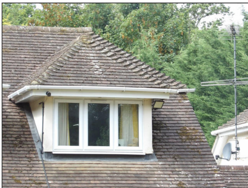
Figure 9. Example flush lead flashing. Norfolk Lodge, Park Lane, Finchampstead. 28.08.26
