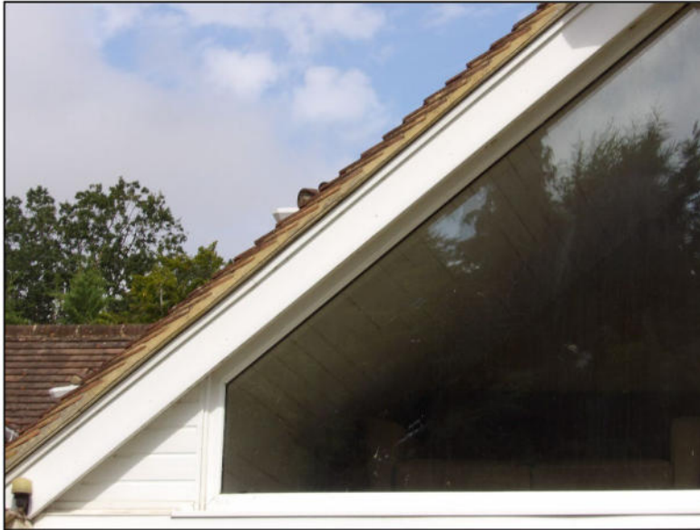
Figure 11. Well-fitting hanging tiles. Norfolk Lodge, Park Lane, Finchampstead. 28.08.26
