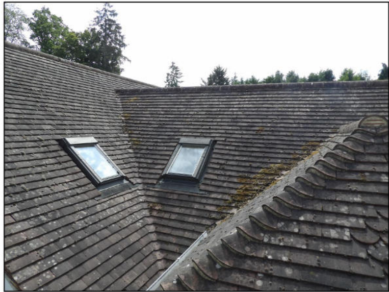
Figure 6. Example missing mortar from ridge tiles. Norfolk Lodge, Park Lane, Finchampstead. 28.08.26
