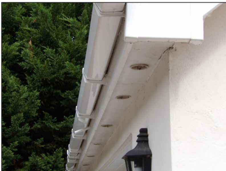
Figure 15. Example sealed soffits/fascias on garage. Norfolk Lodge, Park Lane, Finchampstead. 28.08.26
