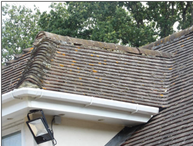
Figure 6. Example missing mortar from ridge tiles. Norfolk Lodge, Park Lane, Finchampstead. 28.08.26
