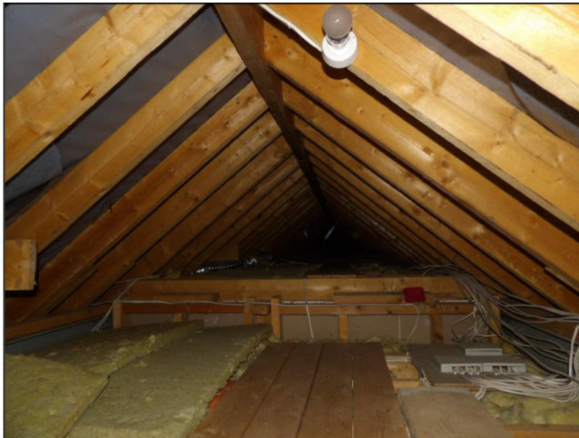
Figure 16. Loft space. Norfolk Lodge, Park Lane, Finchampstead. 28.08.26
