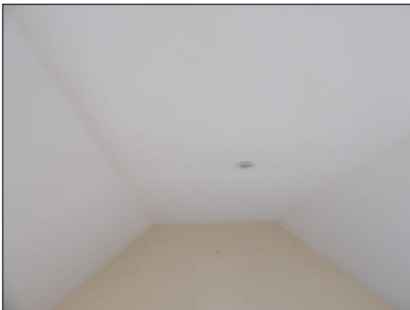
Figure 17. Internal view of first floor of garage. Norfolk Lodge, Park Lane, Finchampstead. 28.08.26
