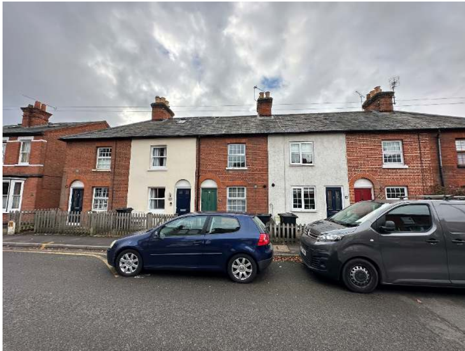
STREET VIEW OF 25, LANGBOROUGH ROAD
