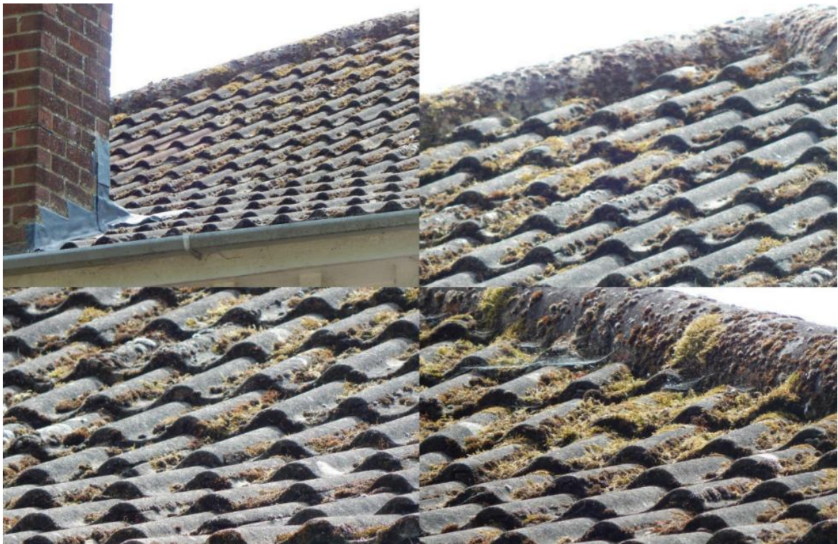
Image 5 – Close view of main roof coverings to demonstrate condition throughout
