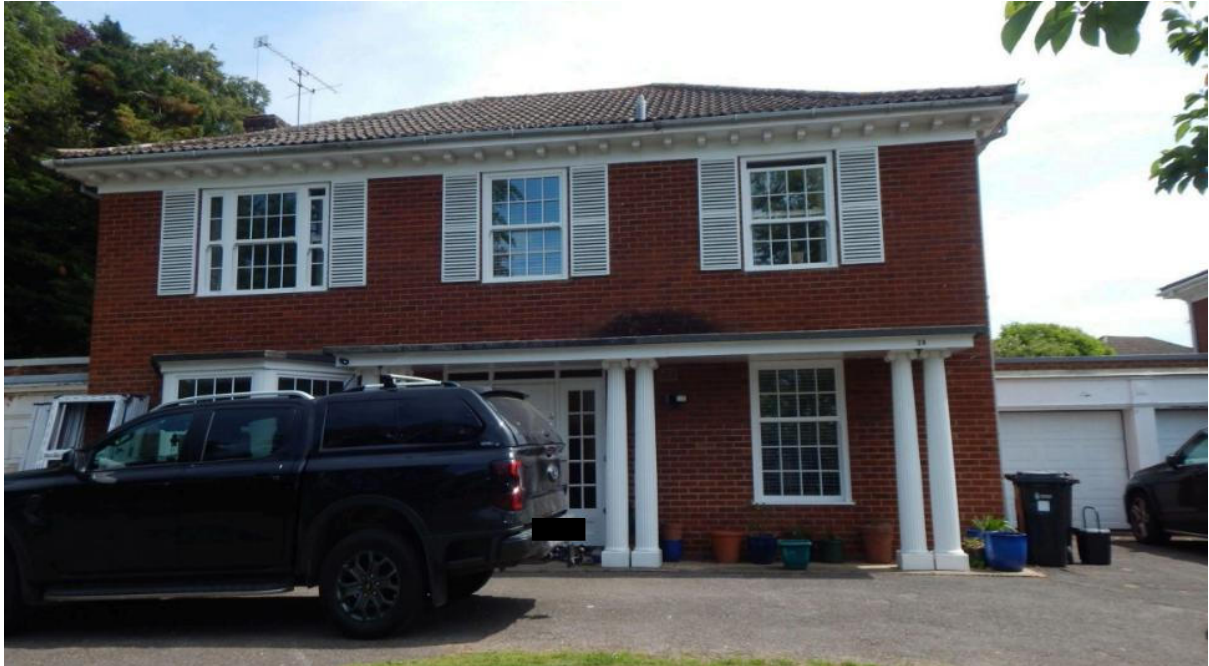
Image 1 – West facing elevation of the property
