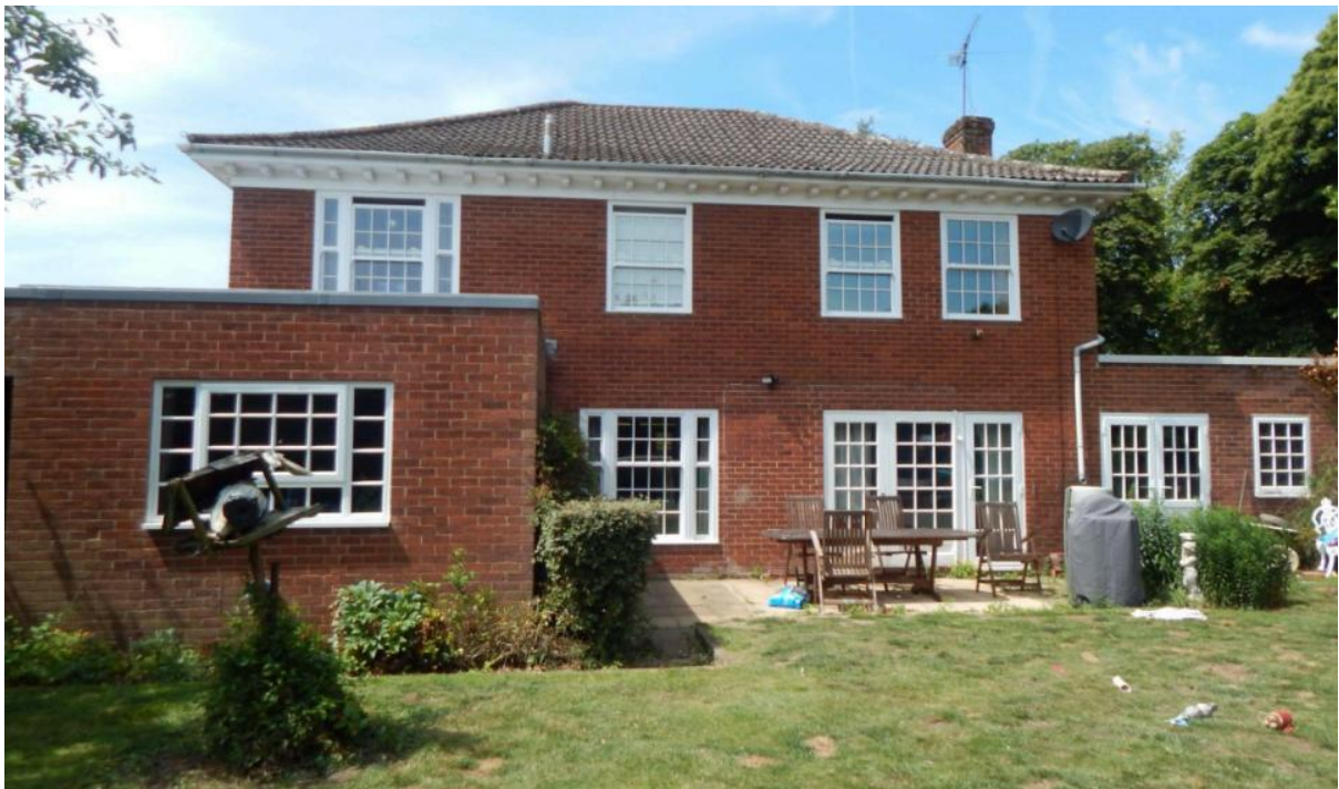
Image 2 – East facing elevation of the property
