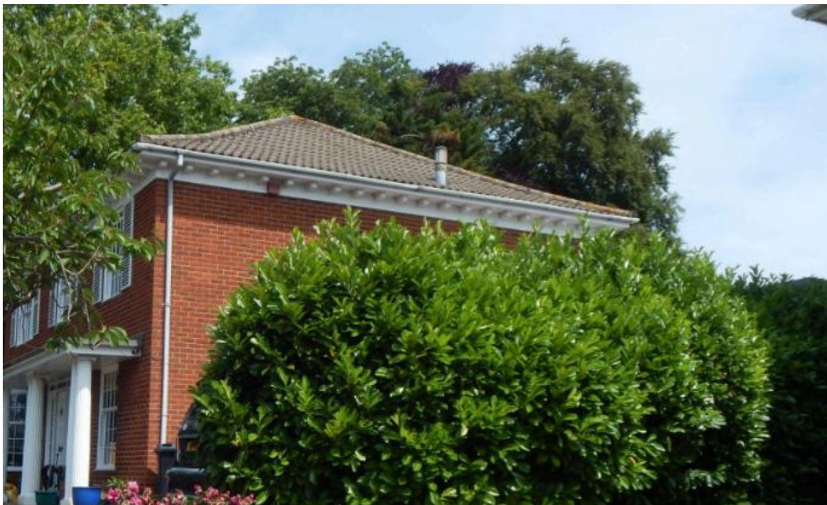
Image 4 - South facing elevation of the property
