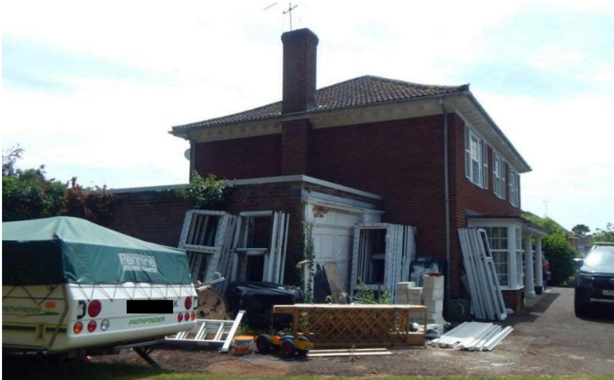
Image 3 – North facing elevation of the property
