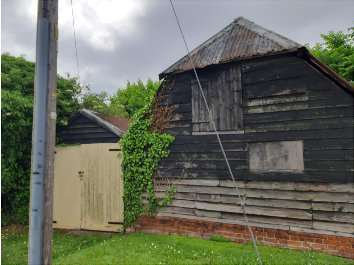
Front (north) elevation of garage (left) and barn
