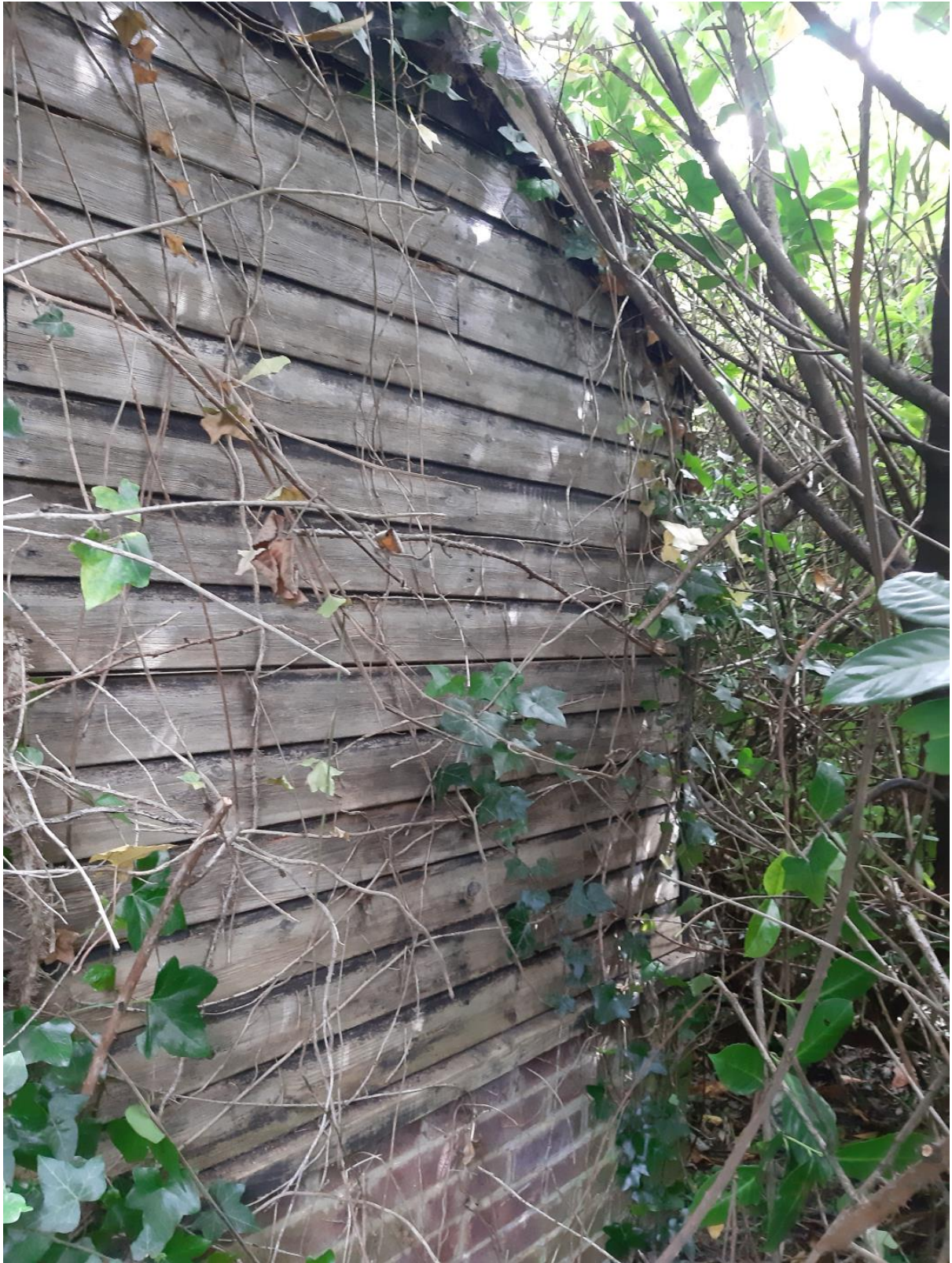
Detail of boarding at rear (south) elevation of garage
