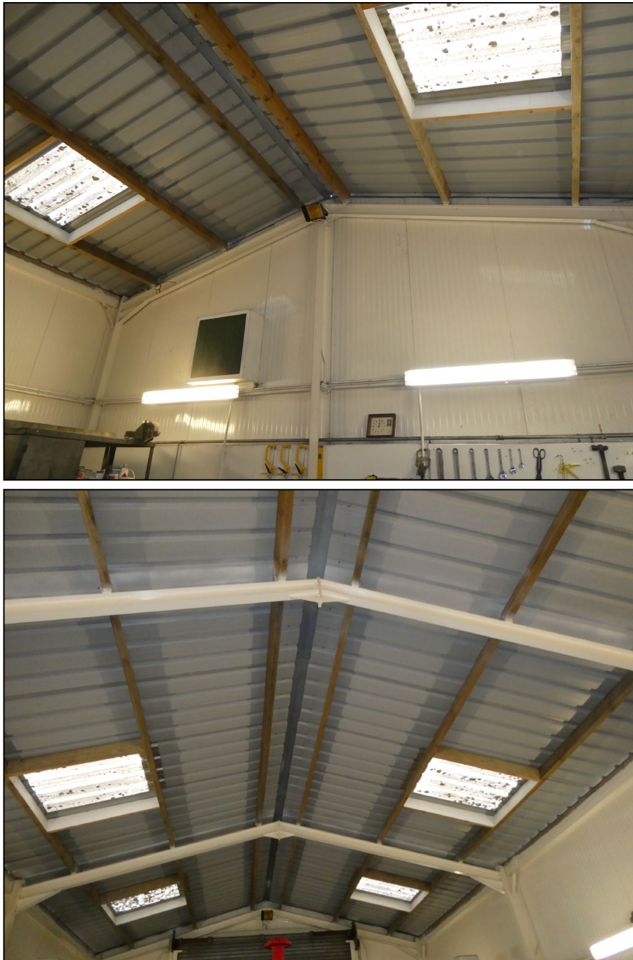
Figure 7. Internal view of workshop at Springfields, Trowes Lane, Swallowfield. 01.02.23
