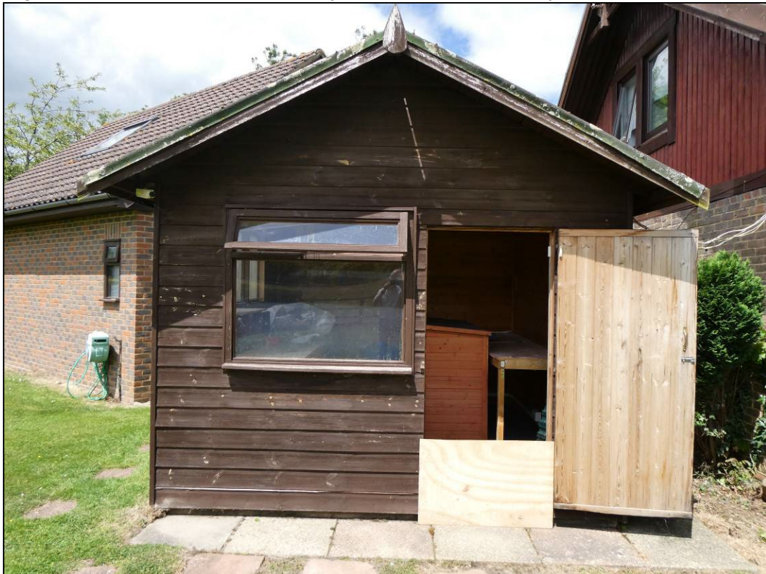
Figure 14. Wooden shed. West Greylake, Part Lane, Riseley. 06.05.24
