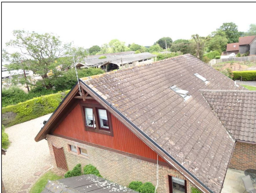
Figure 6. Example of roof tiles. West Greylake, Part Lane, Riseley. 06.05.24
