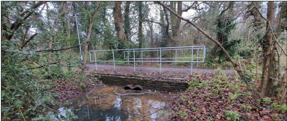
Figure 1. Culvert at NGR: SU 79845 69227 that is proposed to be replaced with a footbridge.
