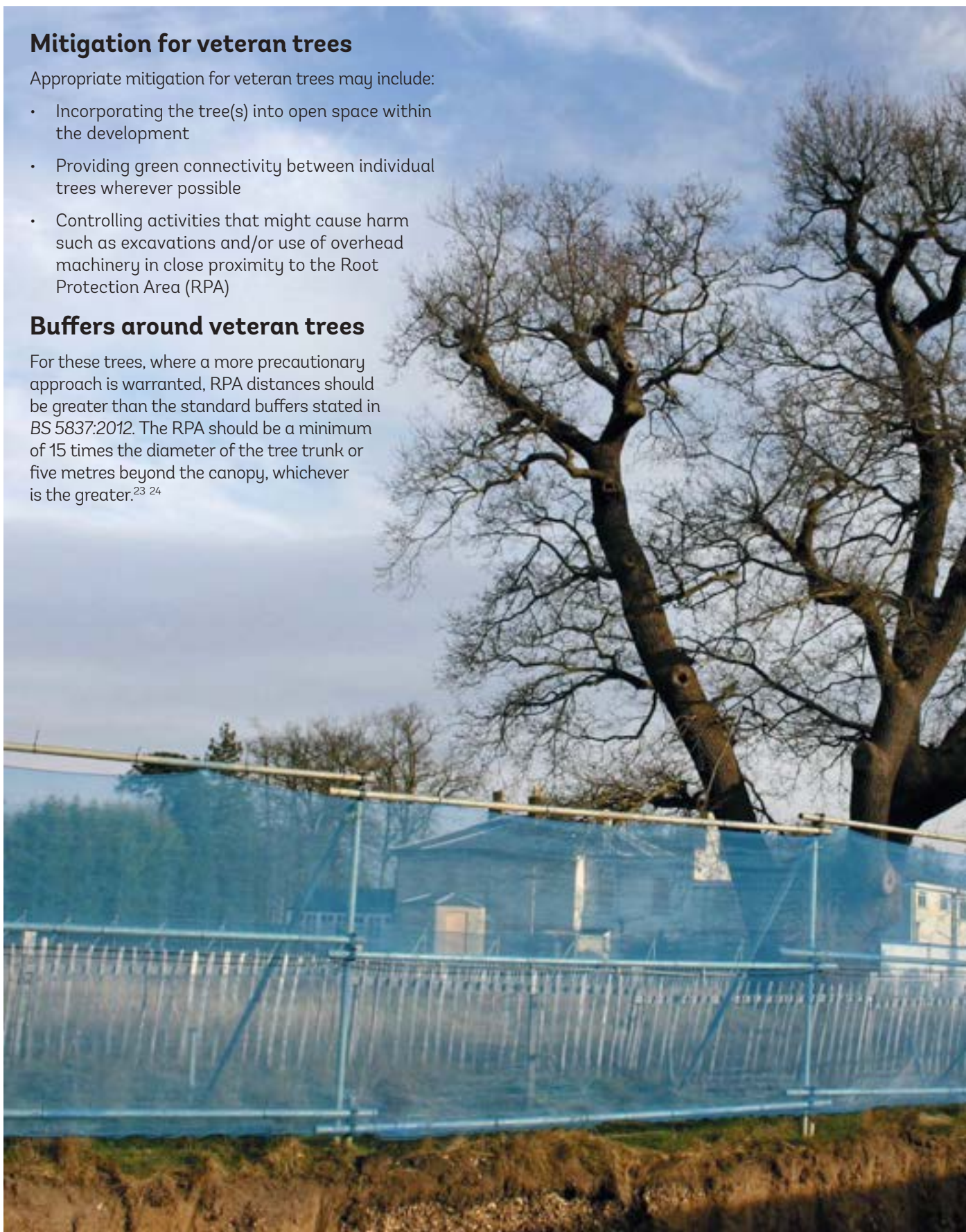
Excavation close to veteran tree
