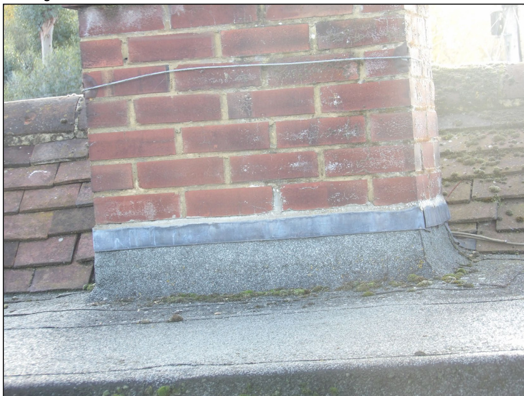
Figure 7. Example flush lead flashing/bitumen felt on chimney stack. 73 Oxford Road, Wokingham. 04.11.25
