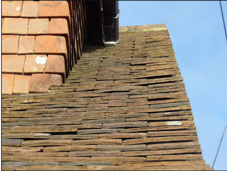
Figure 5. Example raised roof tiles on front elevation. 73 Oxford Road, Wokingham. 04.11.25
