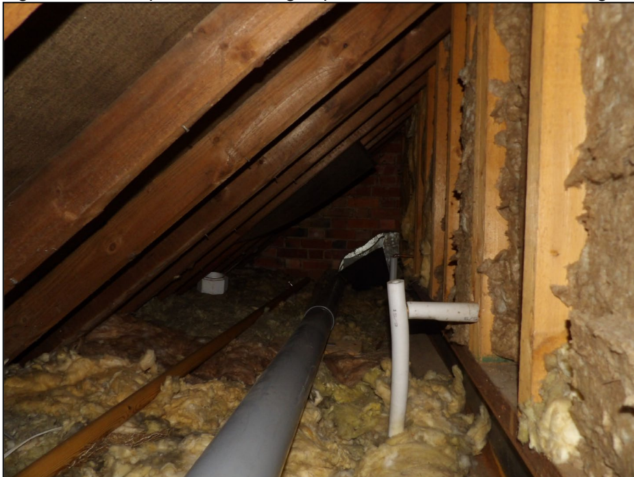
Figure 11. Example eaves storage spaces. 73 Oxford Road, Wokingham. 04.11.25
