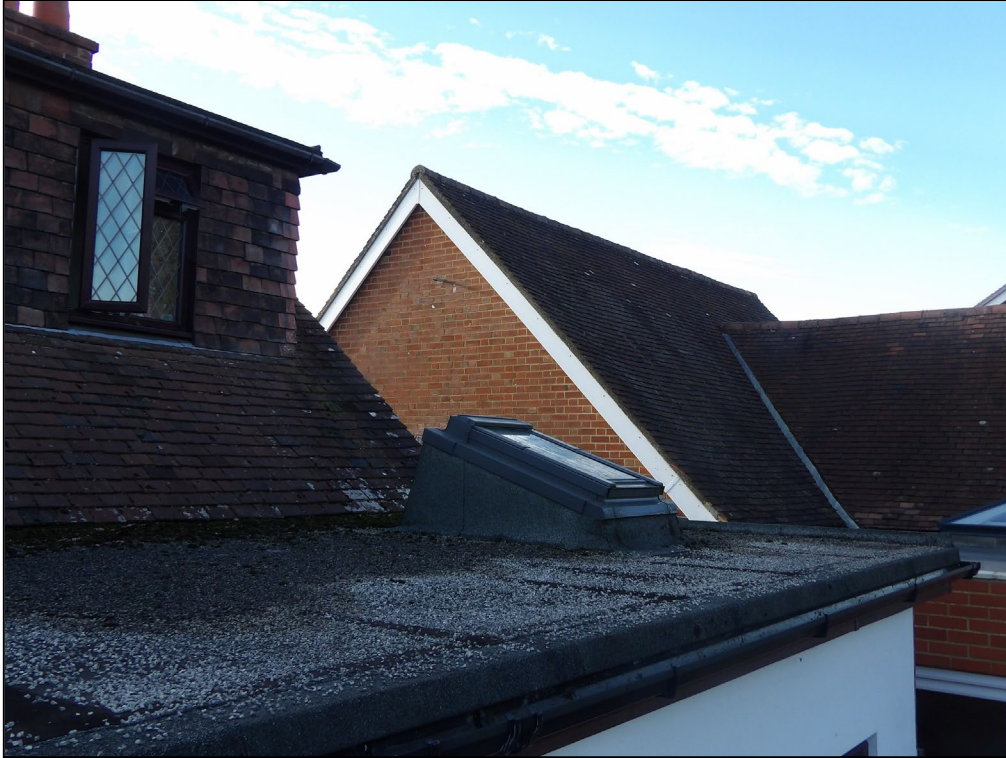
Figure 8. Example well fitted bitumen felt on rear, single storey extension. 73 Oxford Road, Wokingham. 04.11.25
