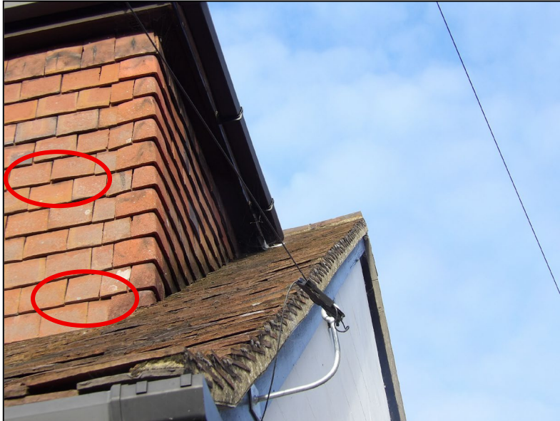
Figure 10. Example moved hanging tiles on dormers windows leaving gaps. 73 Oxford Road, Wokingham. 04.11.25
