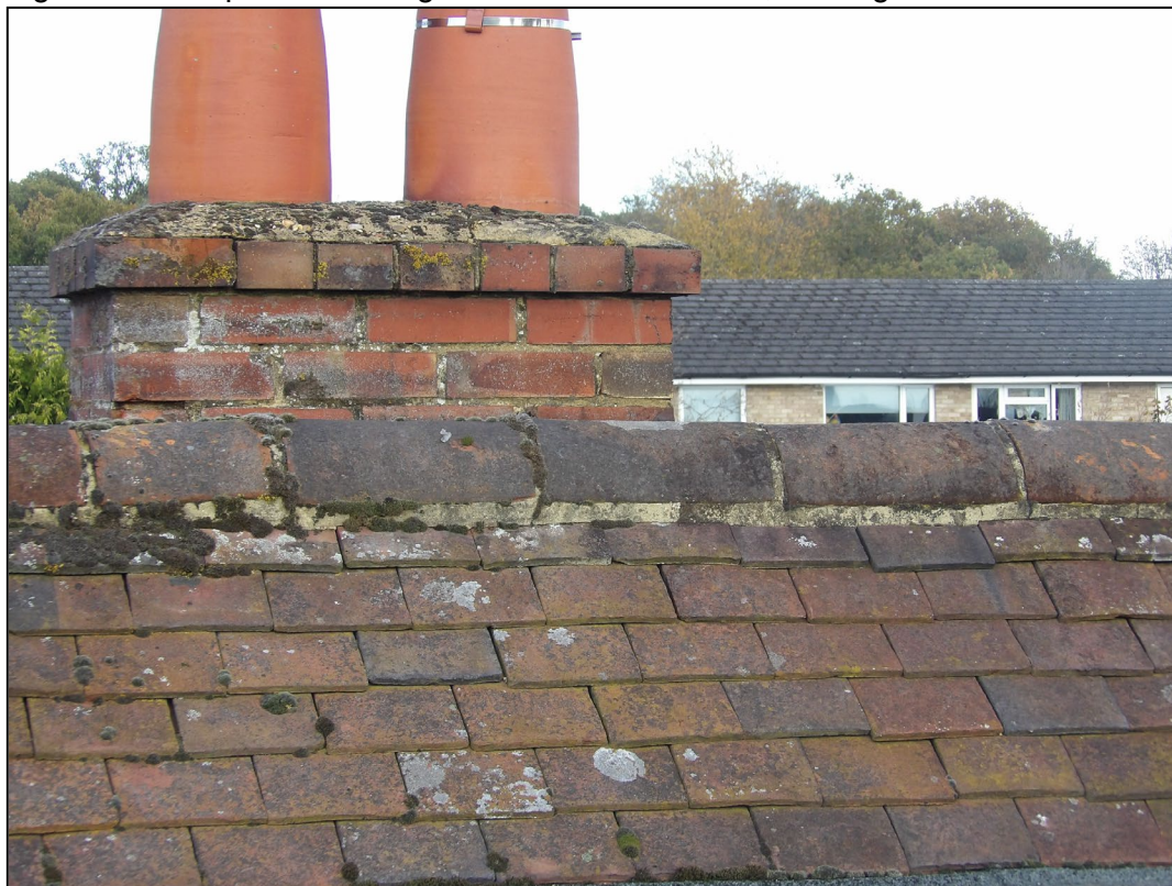
Figure 6. Example sealed ridge tiles. 73 Oxford Road, Wokingham. 04.11.25
