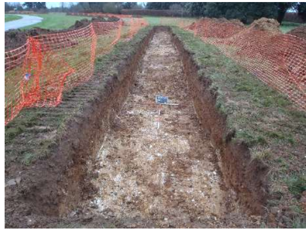
Plate 16 North facing shot of Trench 4
