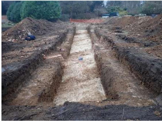
Plate 85 North facing shot of trench 23
