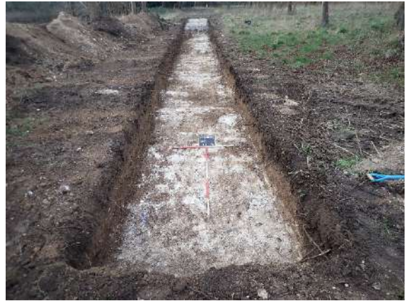
Plate 76 Southwest facing shot of trench 19
