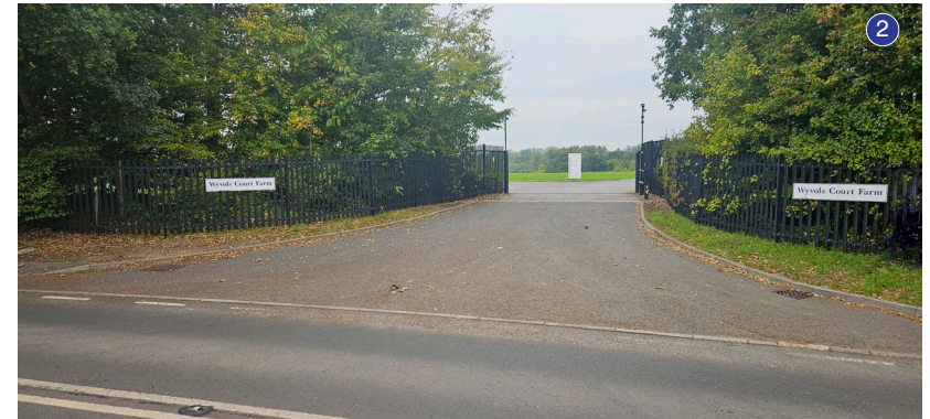
2.02 ~ Security fencing and gate at site access
