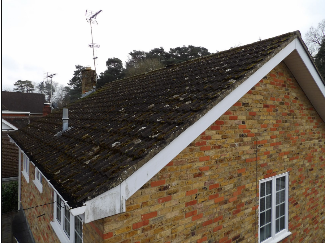
Figure 5. Example of sealed verges. 216b Nine Mile Ride, Wokingham. 21.01.25
