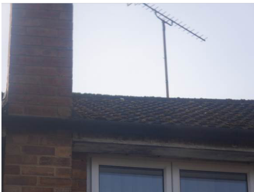
Photograph 5. Flat roof and ridge tiles intact throughout, chimney lead flashing flat.
