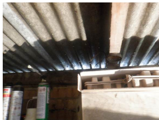
Photograph 12. Roof sheets with multiple gaps causing draughts.
