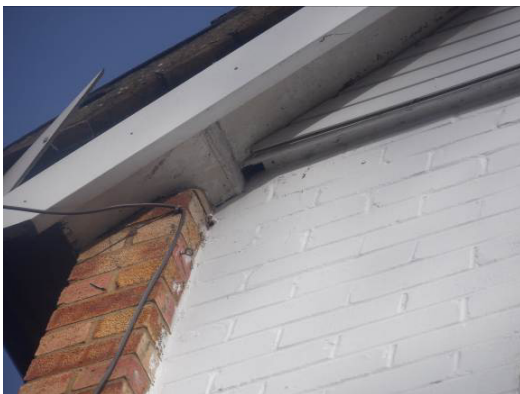
Photograph 9. Small gap beneath front gable uPVC cladding.
