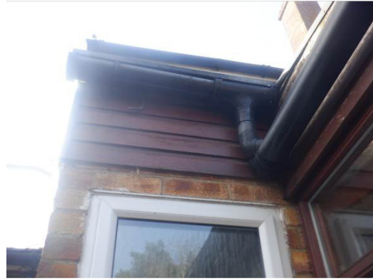
Photograph 8. Soffits and cladding tight to brickwork (northern elevation).
