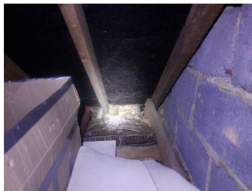
Photograph 16. Eaves filled with fibreglass insulation.
