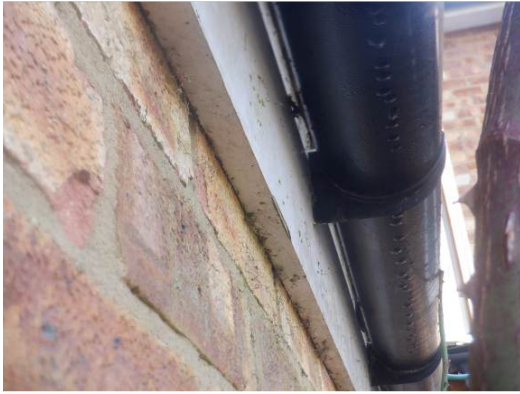
Photograph 7. Soffits tight to brickwork throughout.
