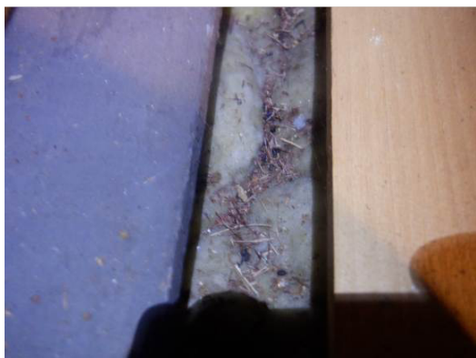
Photograph 15. Fibreglass insulation on part-boarded floor.
