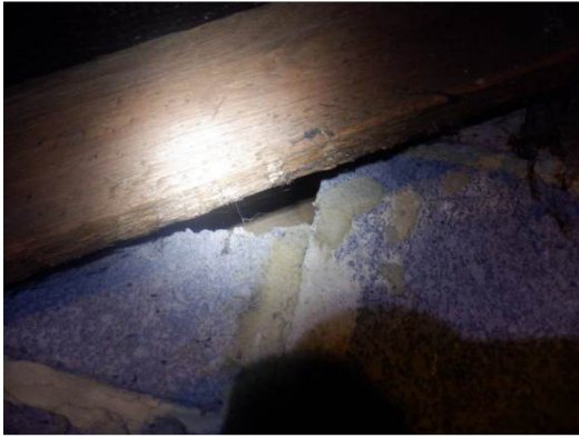
Photograph 17. Blockwork gables with gaps behind end rafters.
