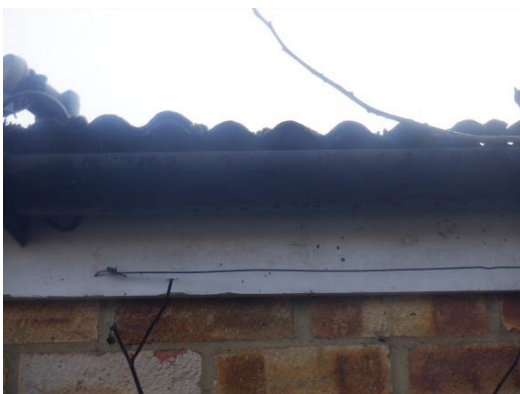
Photograph 11. Timber soffits tight to brickwork on garage.
