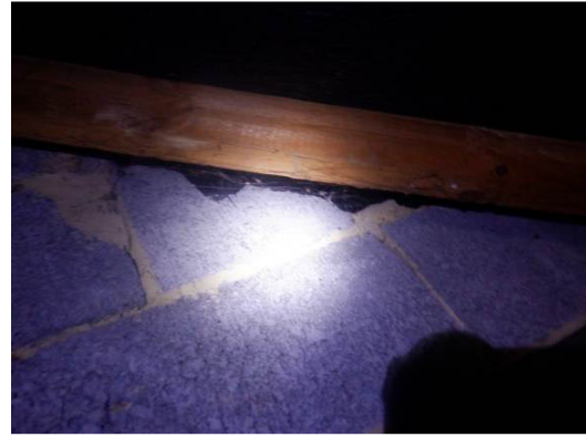
Photograph 18. Blockwork gables with gaps behind end rafters.
