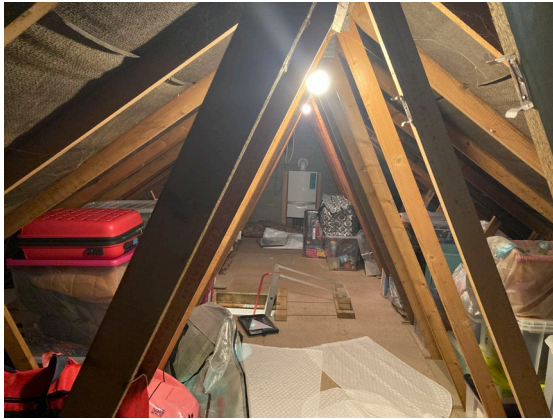
Photograph 8. The roof void showing the trussed rafters.
