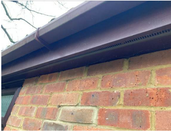
Photograph 5. Intact soffits tightly fitted to the brickwork.
