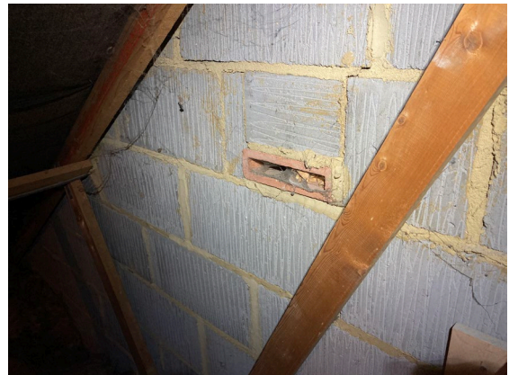
Photograph 11. The vent bricks in the side (north east facing) gable.
