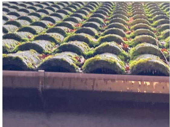
Photograph 4. Insect mesh filling tile ends above the gutter
