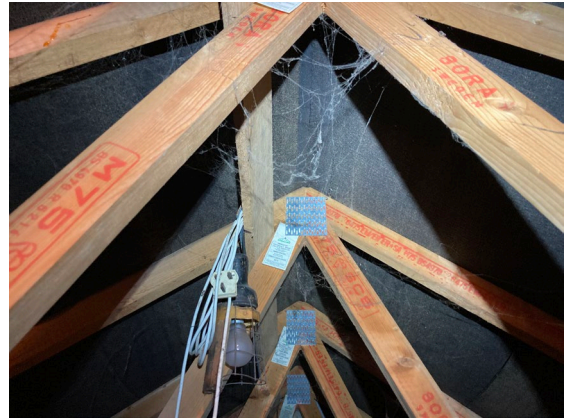
Photograph 9. The intact bitumen felt cobwebbed at the ridge.
