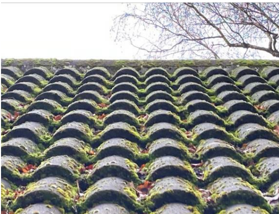
Photograph 3. Tightly fitted pantiles and ridge.
