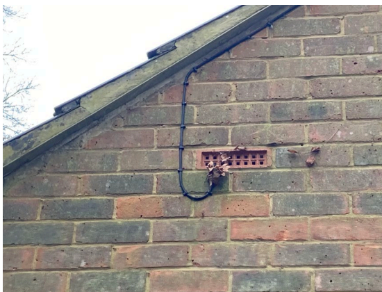
Photograph 7. The vent bricks and intact verge mortar on the side gable
