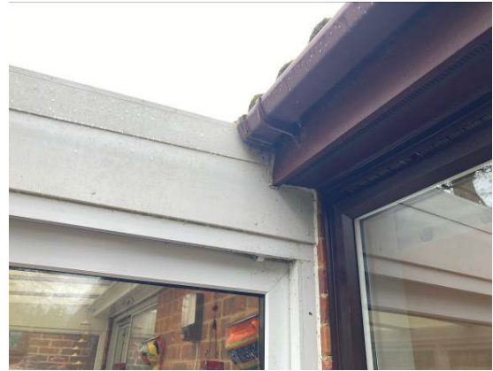
Photograph 6. The conservatory sealed to the soffits.
