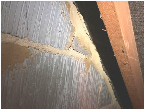
Photograph 10. The felt sealed to the blockwork at the gable end and party wall.
