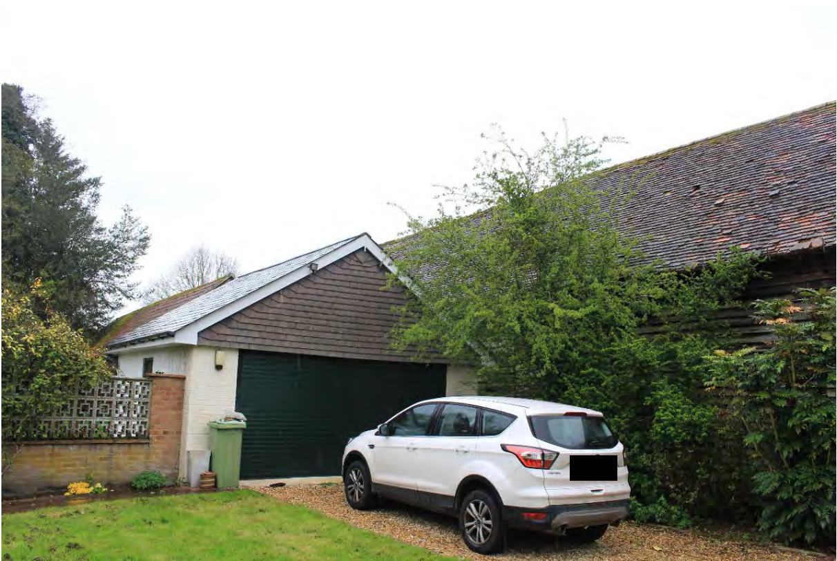
Image EDP A1.8: East facing view from the modern post-1970s cottage towards its associated modern garage, adjacent to the listed barn of Pearce's Farm ( 1118118 ). The modern garage is illustrated to be of the same unsympathetic design and use of modern materials, not in keeping with the character of Pearce's Farmhouse ( 1319115 ) or its associated barn ( 1118118 ).
