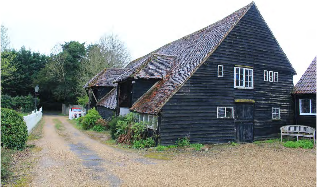
Image EDP A1.11: West-facing view from Pearce's Farm's farmyard. View of listed barn ( 1118118 ), illustrating the vernacular architectural style of the barn and its later 20 th century window encasement additions on its east side.
