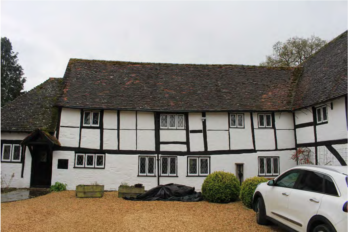
Image EDP A1.2: South-facing view of Pearce's Farmhouse ( 1319115 ) from centre of Pearce's Farm's farmyard. Appearance of the farmhouse shown with views towards farmyard. Later 20 th century window casements shown also.
