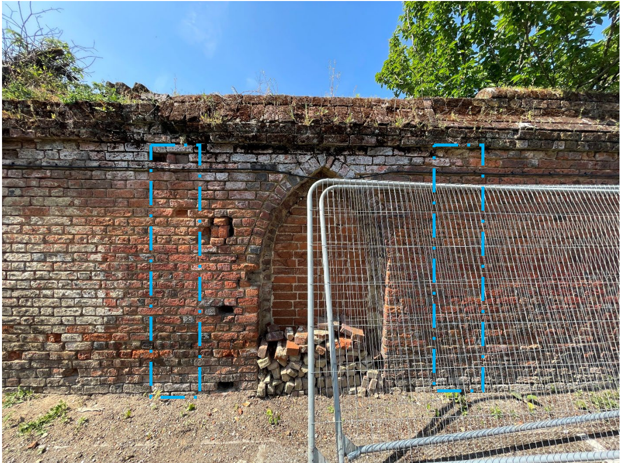
Photograph 5 – Suggested buttress locations (or similar to other side if reverse-buttress used)
