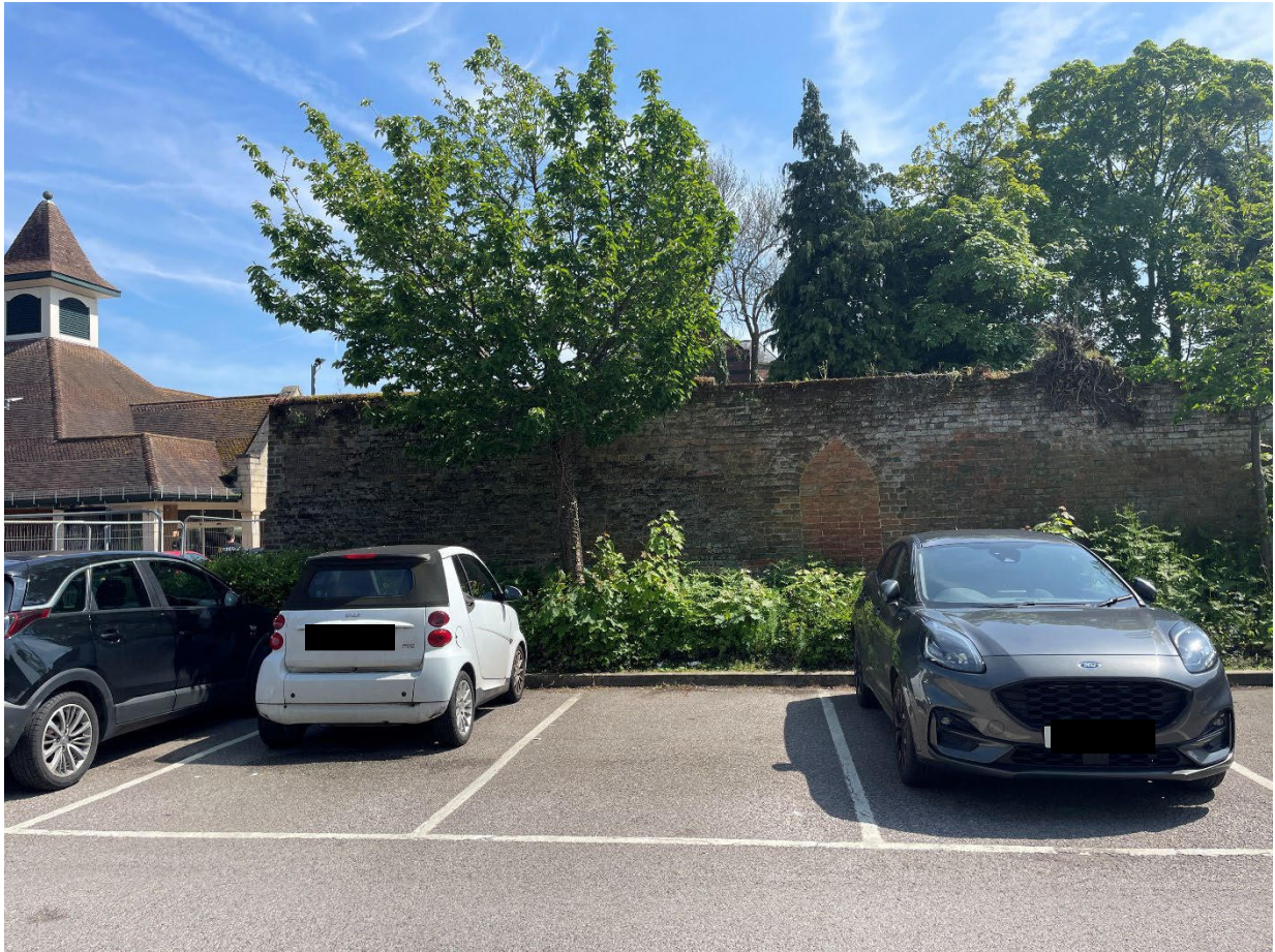
Photograph 1 – Elevation from north side of wall
