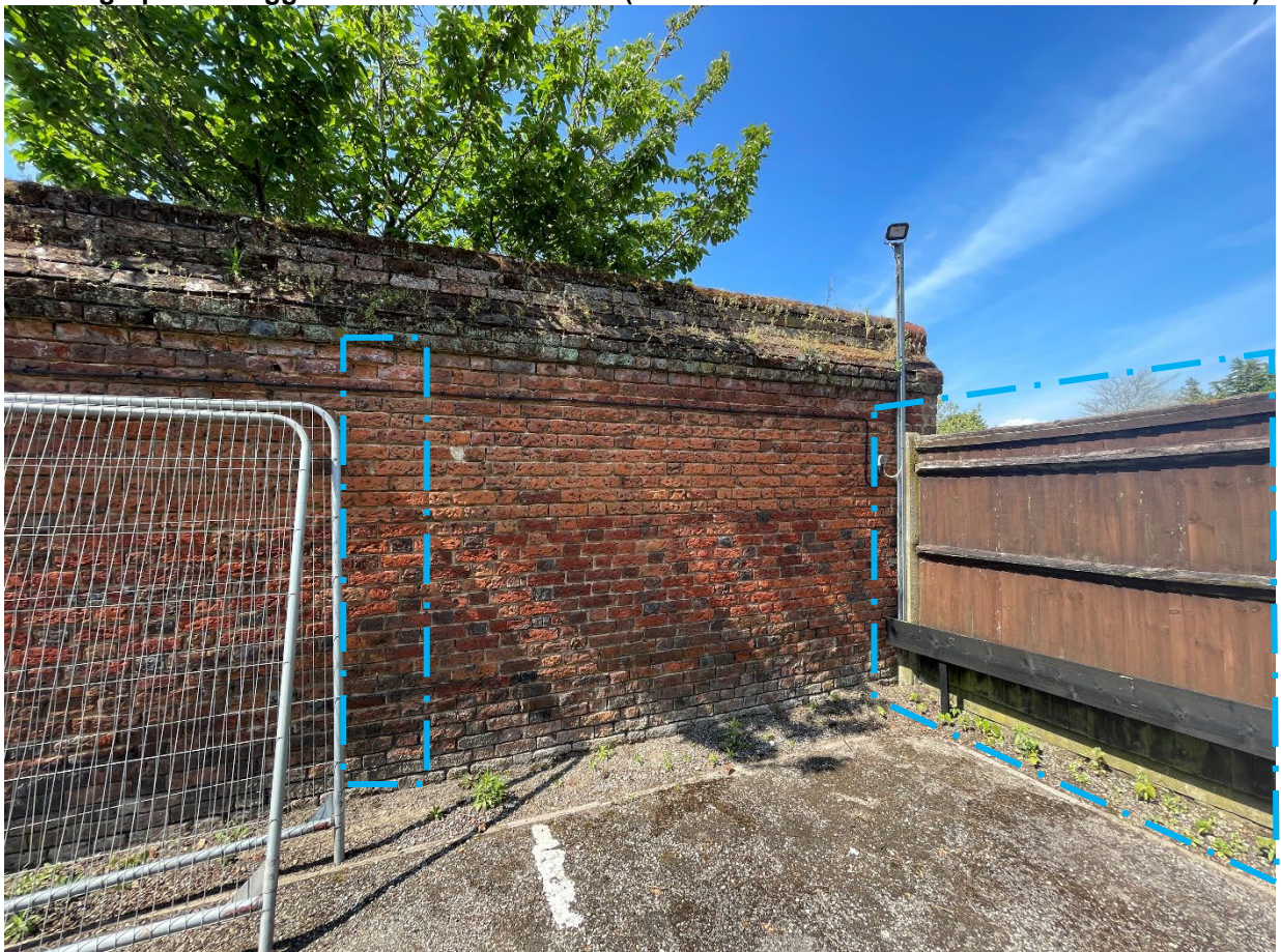
Photograph 6 – Suggested buttress locations (or similar to other side if reverse-buttress used)
