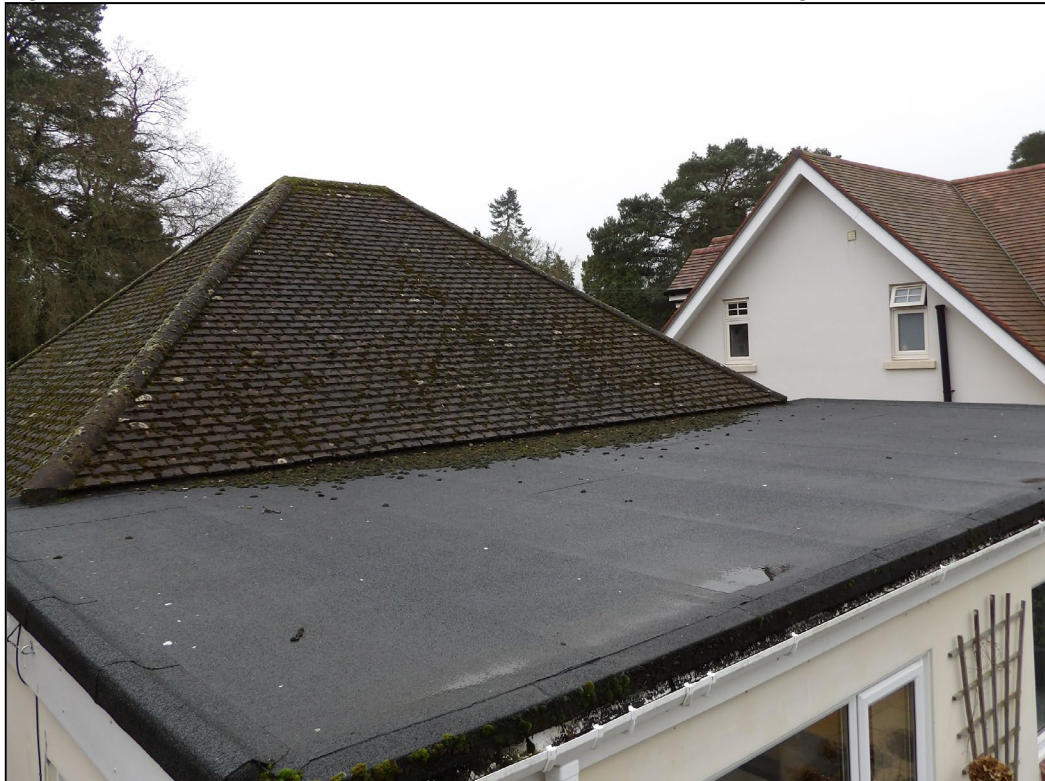
Figure 8. Roof of rear extension. 179A Nine Mile Ride, Wokingham. 10.02.26
