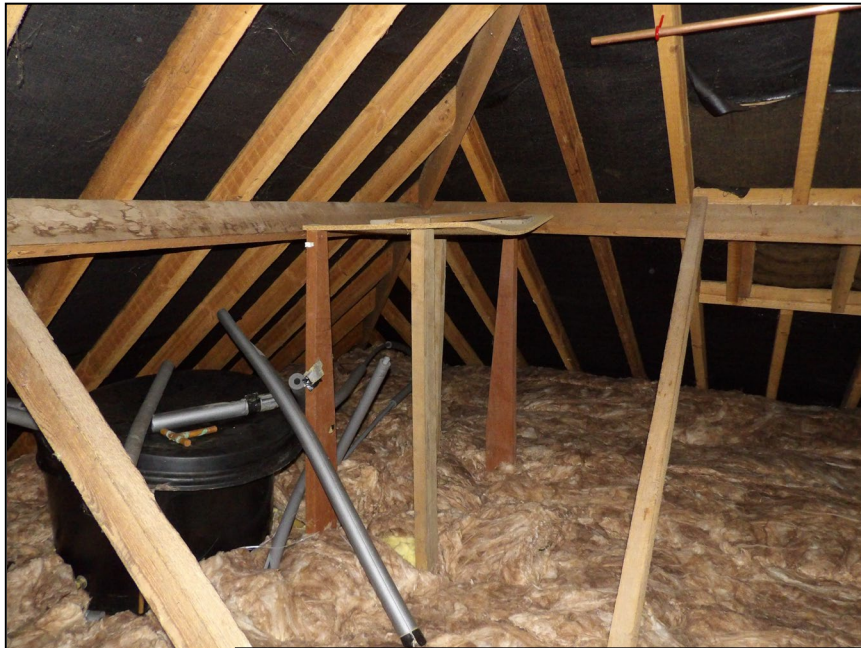
Figure 9. Example of loft space and bitumen lining to roof tiles. 179A Nine Mile Ride, Wokingham. 10.02.26
