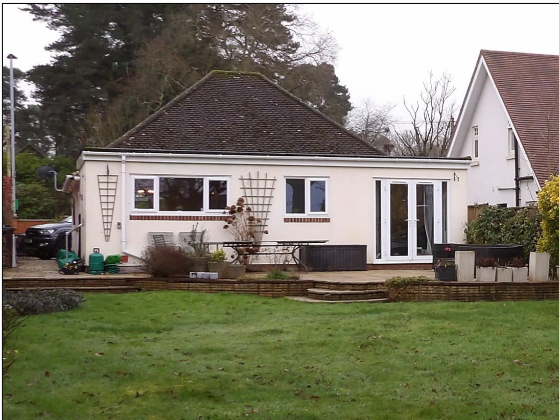
Figure 4. Rear view of property. 179A Nine Mile Ride, Wokingham. 10.02.26
