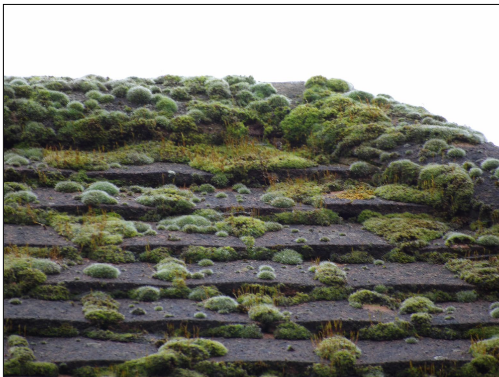
Figure 6. Example of sealed ridge/hip tiles. 179A Nine Mile Ride, Wokingham. 10.02.26
