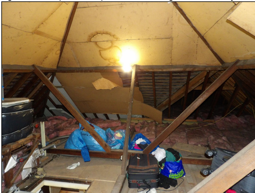
Figure 9. Example of loft space. 108 Reading Road, Woodley. 10.01.25
