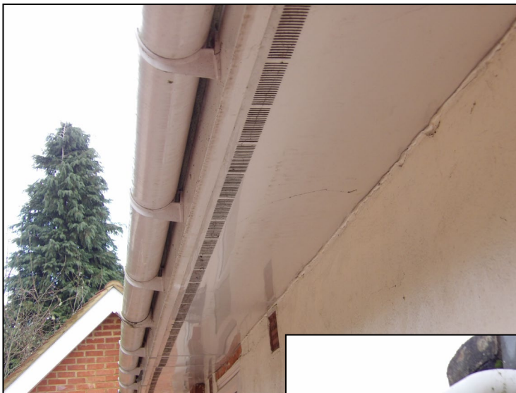
Figure 8. Example sealed uPVC soffits and fascias. 108 Reading Road, Woodley. 10.01.25
