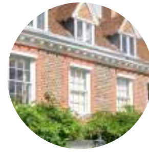
Brick Quoin Detailing & Clay Tile Roof
