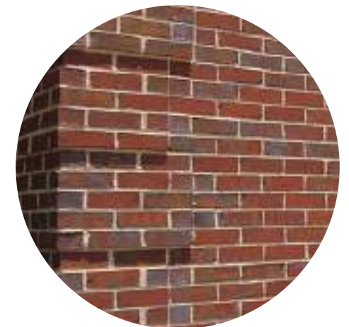
Brick Banding and Quoin Detailing
