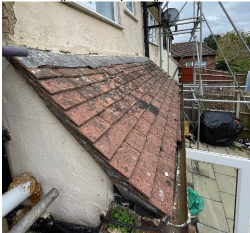
Figure 6. Lower rear extension roof looking east.
