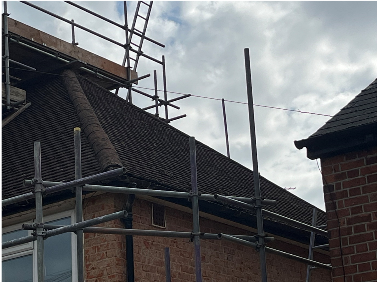
Figure 4. West hip looking southeast.
