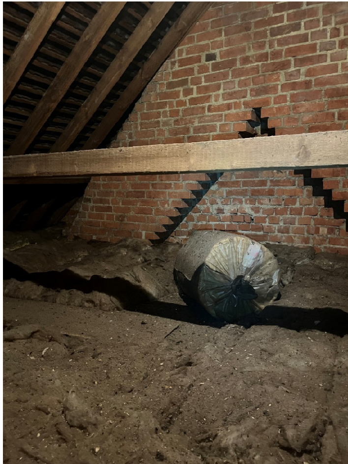
Figure 7. Loft looking northeast.
