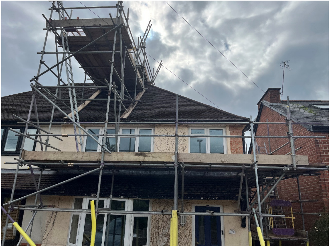
Figure 2. Northern elevations looking south.
