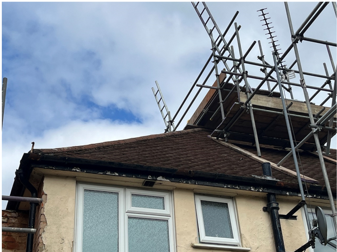
Figure 3. Southern elevation looking northeast.
