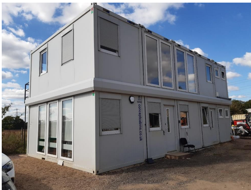
Figure 3: Case Officer Site Visit Photos of Portacabin – Dated 17 th September 2024
