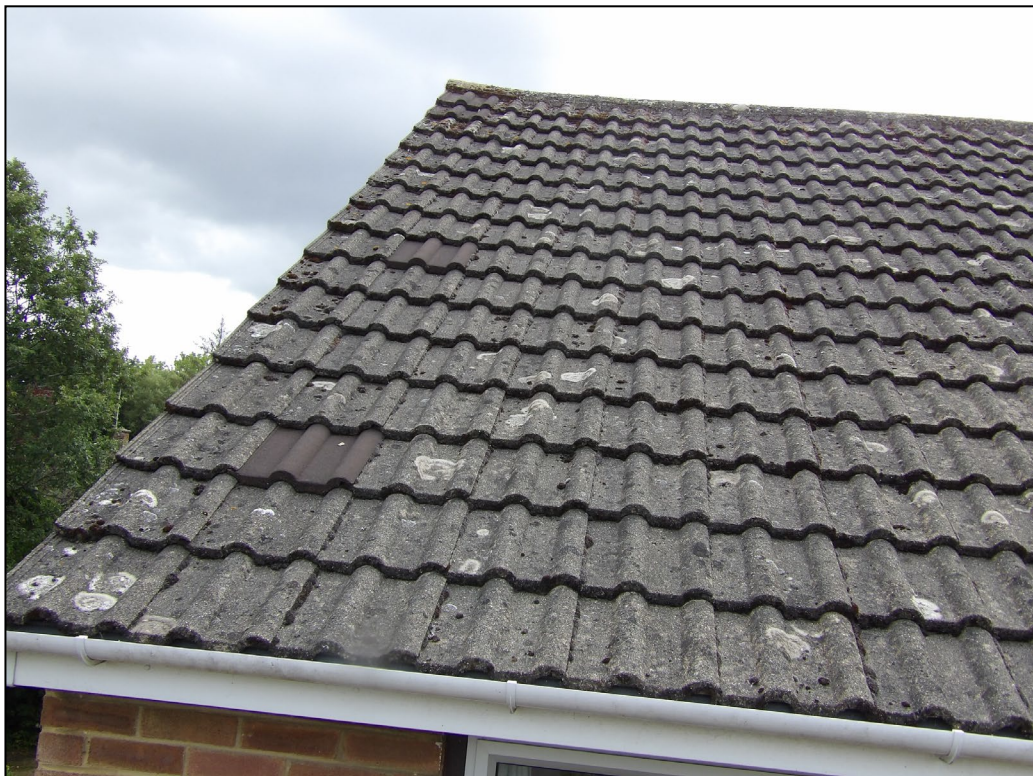
Figure 4. Tightly fitted roof tiles. 155 Old Woosehill Lane, Wokingham. 22.07.25
