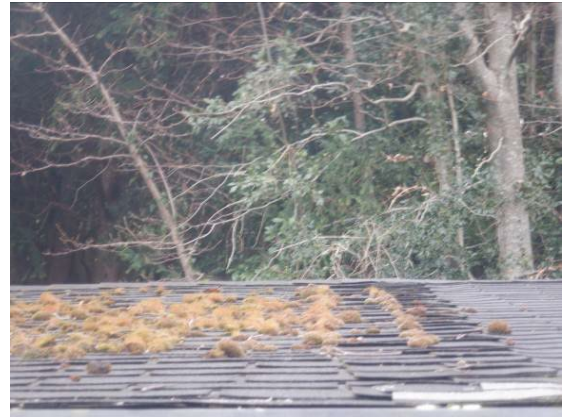
Photograph 6. Bitumen tiles at south western corner with slightly raised tiles but unsuitable for roosting bats.
