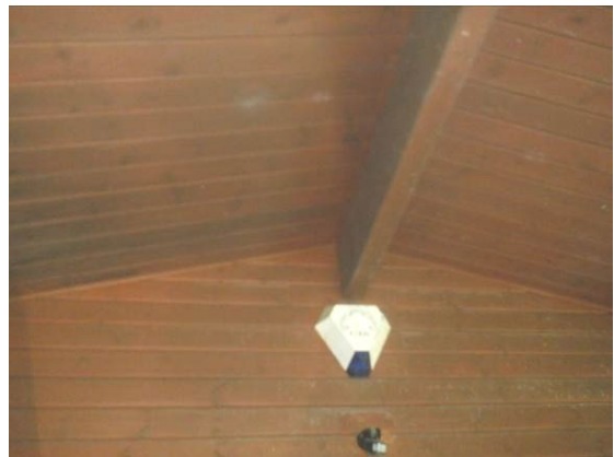
Photograph 4. Tightly fitted timber cladding and underside of roof in front porch at northern end.
