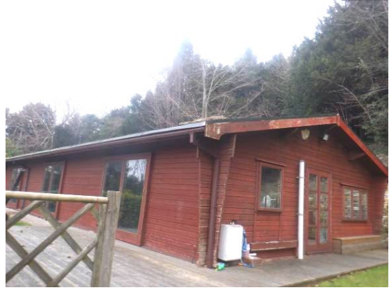
Photograph 2. The property viewed from the south western corner.
