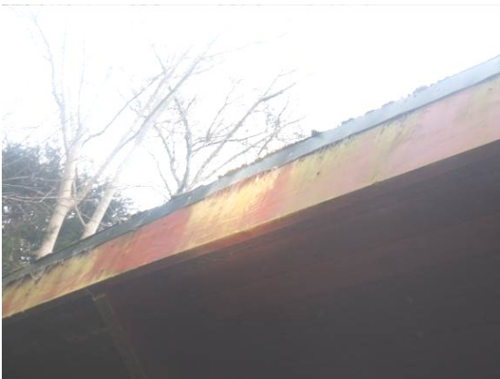
Photograph 3. Slight overlap of roof covering at each gable end – no gaps suitable for roosting bats.
