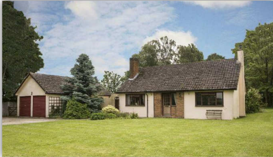
Brandywell House and Garage - Front View
