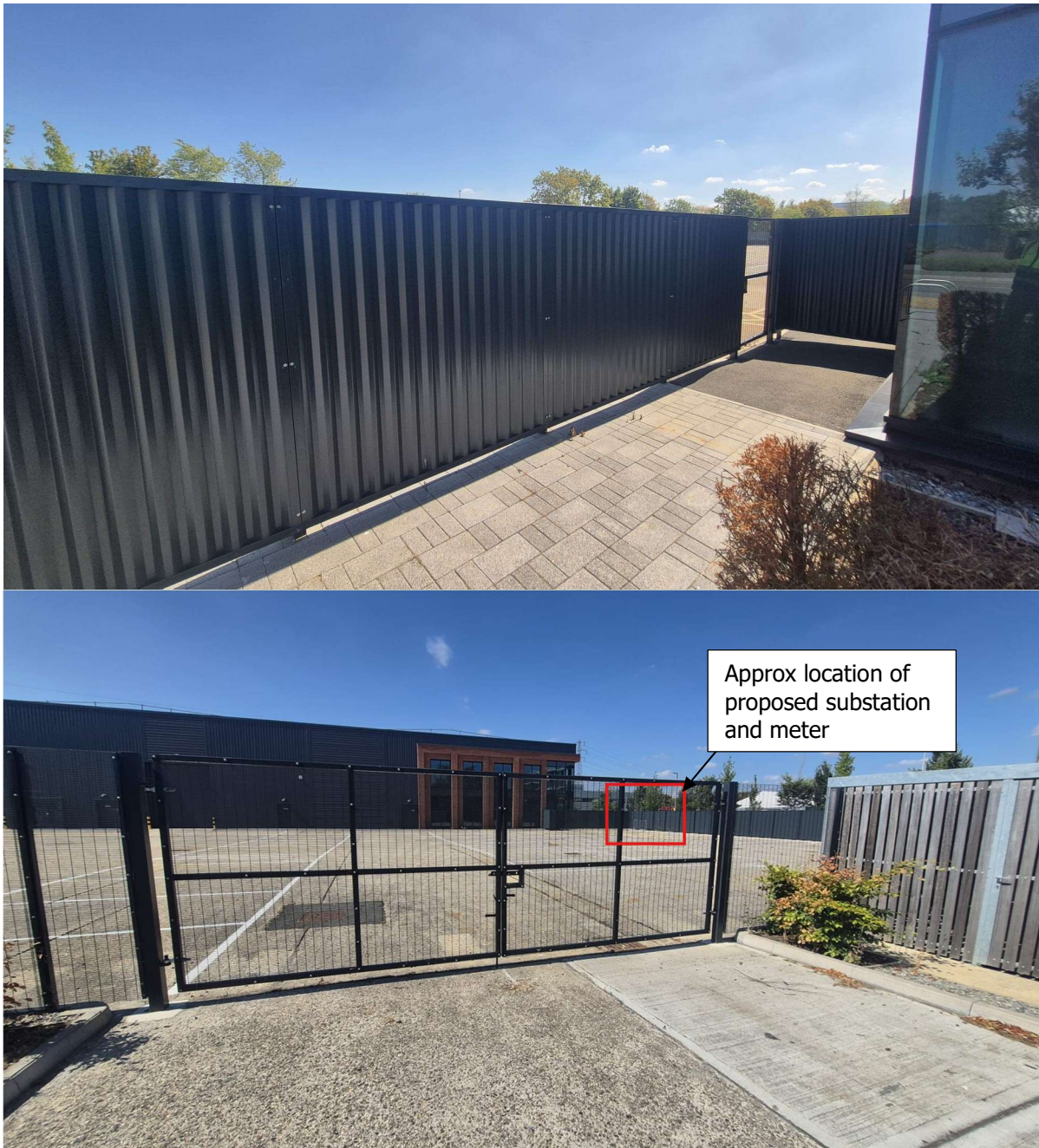
Figure 6: Existing Solid Metal Panel Fencing
