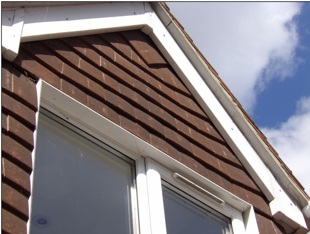
Figure 10. Example close fitting hanging tiles on dormers. 7 Buckhurst Grove, Wokingham. 08.07.25
