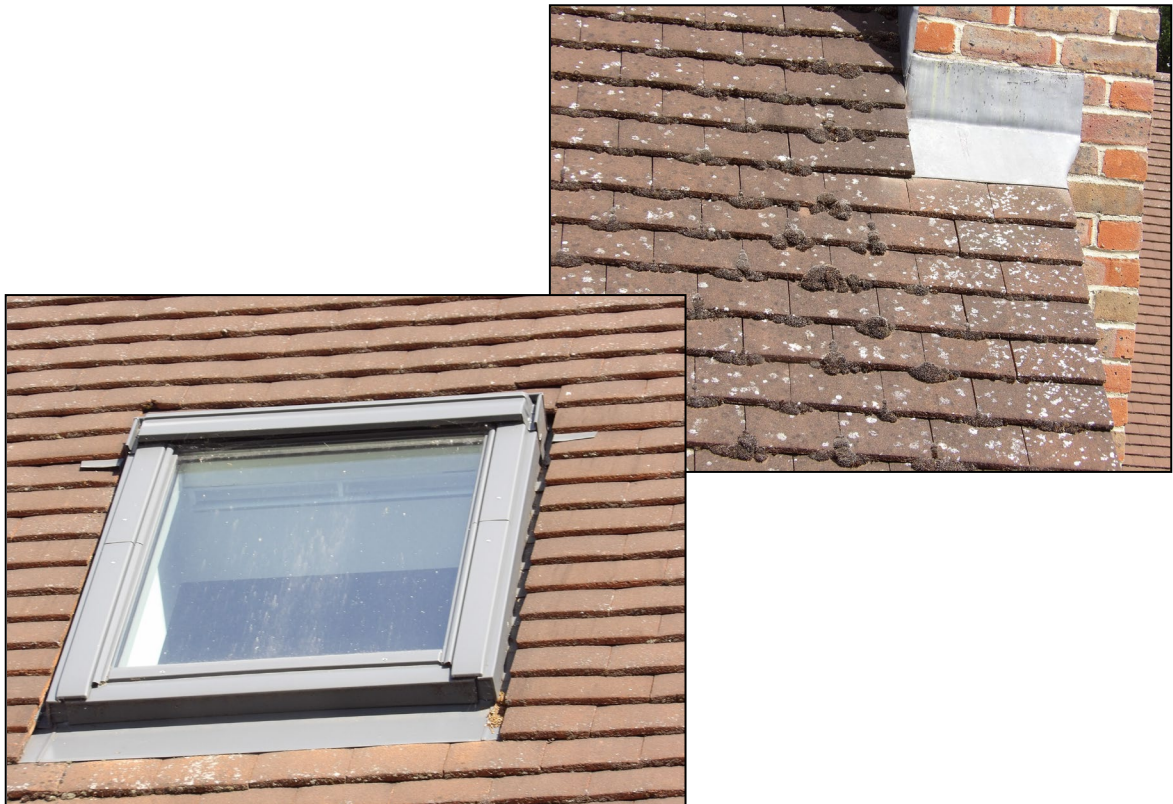
Figure 7. Example flush lead flashing. 7 Buckhurst Grove, Wokingham. 08.07.25
