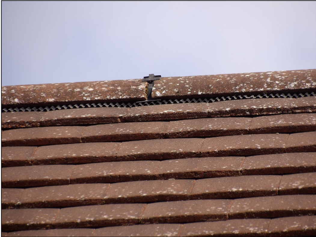
Figure 5. Example of ridge clips. 7 Buckhurst Grove, Wokingham. 08.07.25
