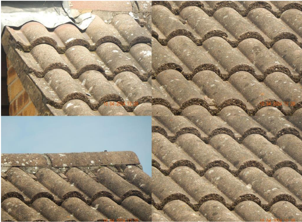
Image 5 – View of the main roof coverings to demonstrate example of condition
