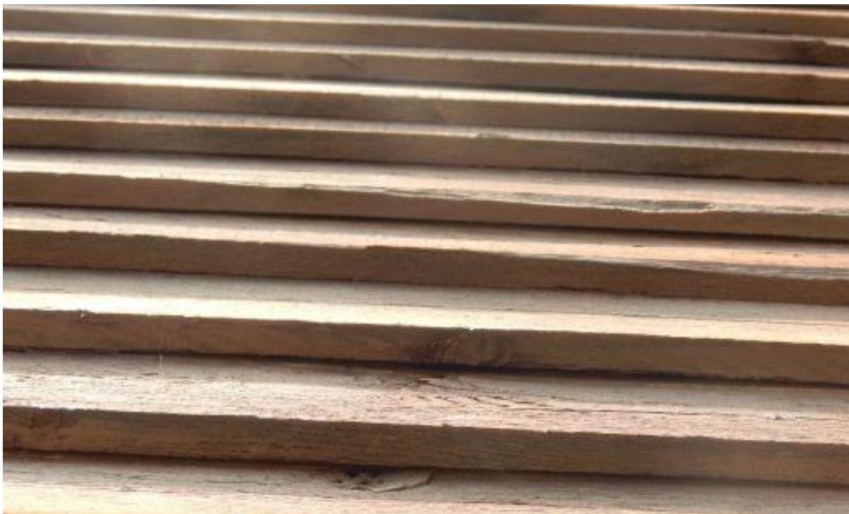
Image 6 – View of the timber cladding coverings to demonstrate example of condition
