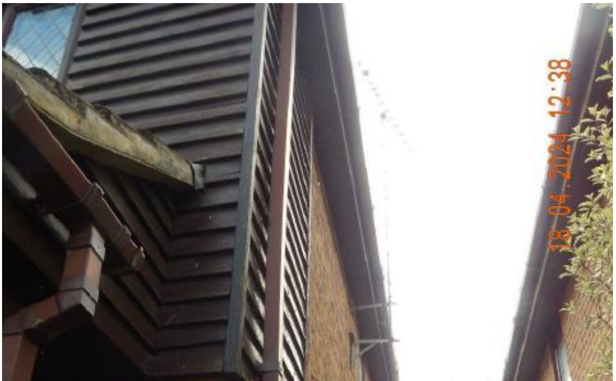
Image 4 – West facing elevation of the property
