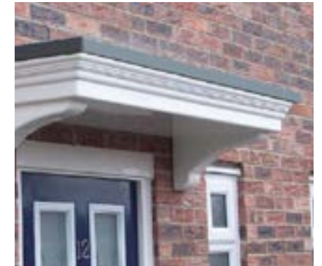
Flat roof porches
