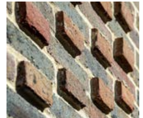
Protruding detailing forms
