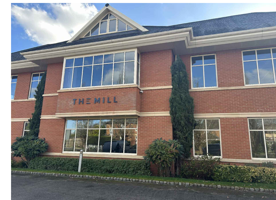
04 EXISTING GROUND FLOOR - EXTERIOR FRONT ELEVATION Photograph
