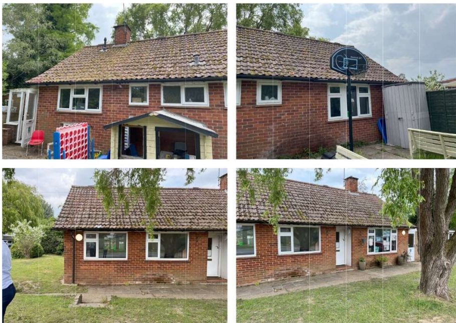
Fig 1 & 2. Existing rear elevation and Fig 3 & 4. Existing frontage of the Bungalow
