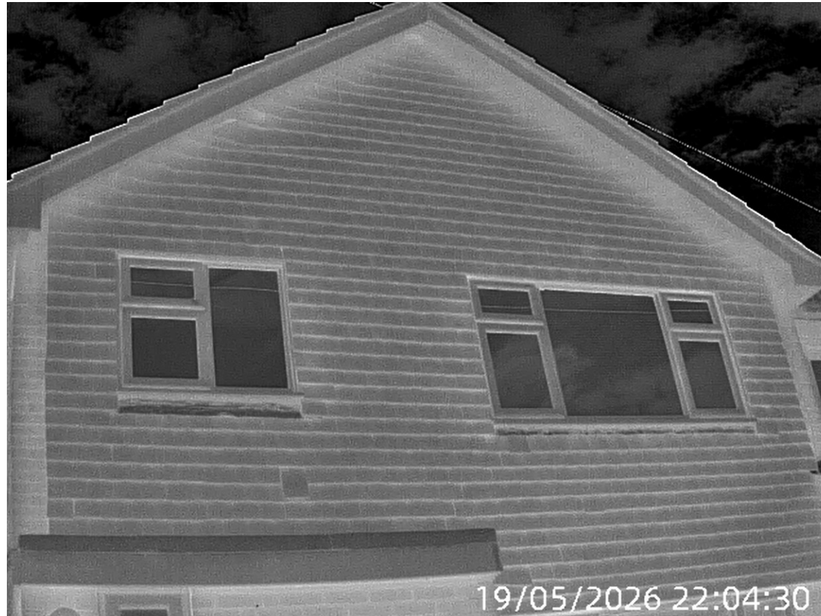
Guide TK612 at Survey Location on 19 h May 2026.
