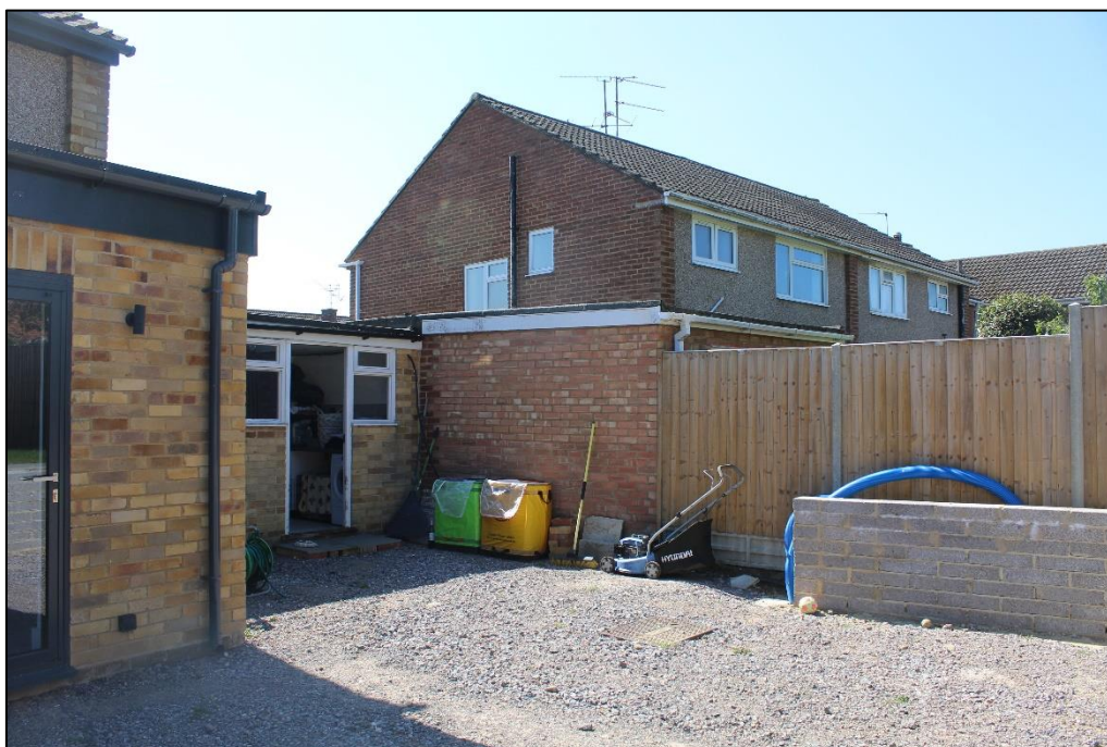
Photograph 4 – Side elevation view of neighbouring property to left-hand boundary
