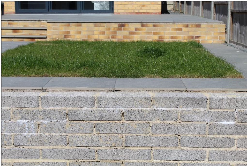
Photograph 3 – Garden area to rear of the property showing the 36cm retaining wall
