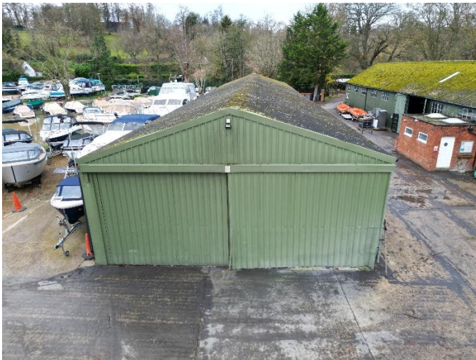
Current Gable End Shed 2
