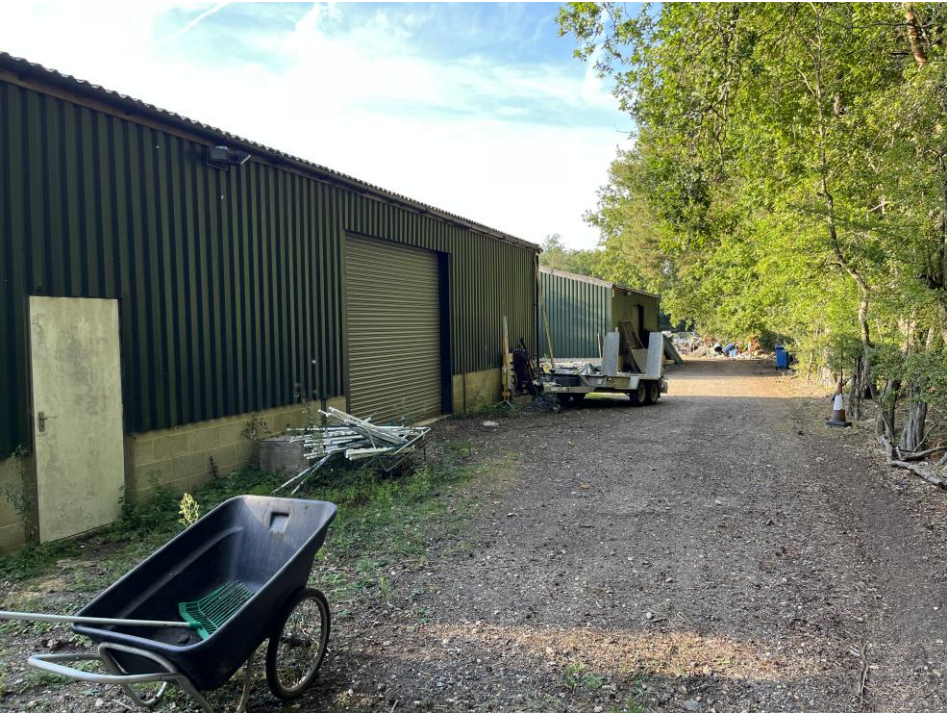
Photo 2 – Showing the buildings and track in the east of the site.
