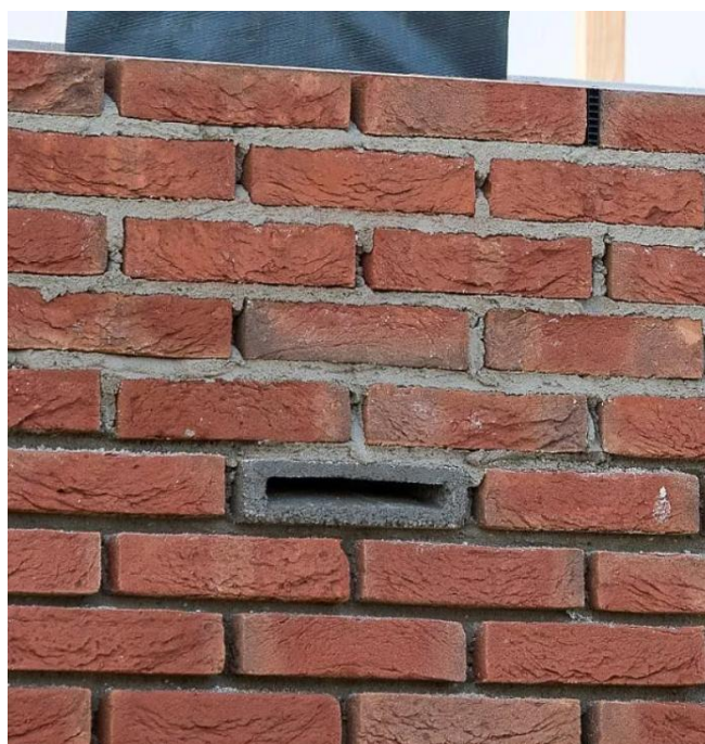
Figure 1. Vivara Pro Build-in Woodstone Bat Box, showing how the box can be integrated into a wall. Source: www.nhbs.com .
