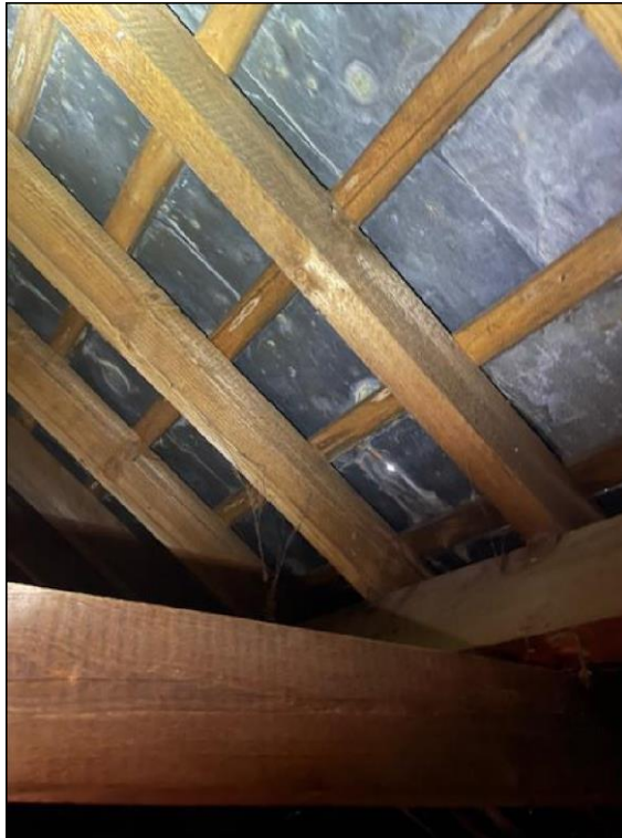
Photograph 13: Loft space no liner straight to slate tiles.
