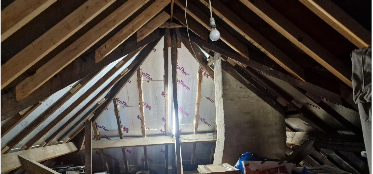
Picture 7: Showing the internal structure of the roof with the insulation between the rafters.
