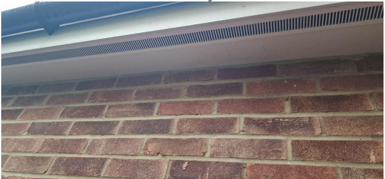
Picture 4: Showing soffit on the single storey extension
