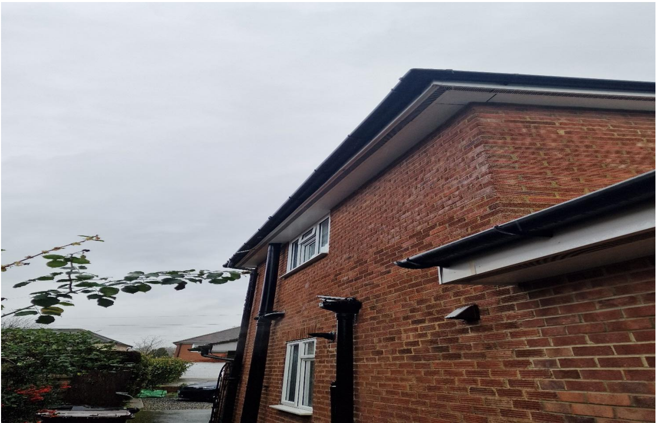
Picture 5: Showing the soffit on the main house
