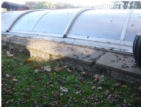
Photograph 9. Covered swimming pool with a patio around the edge.
