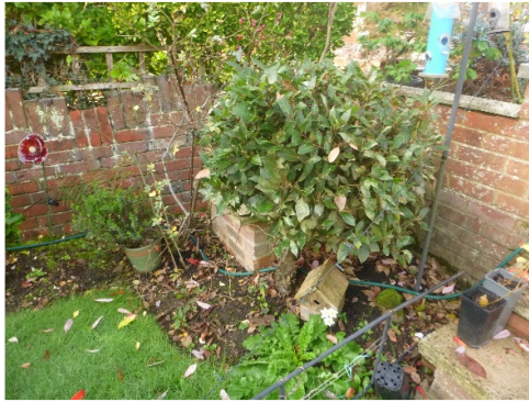
Photograph 7. Wall around the rear garden and patio.
