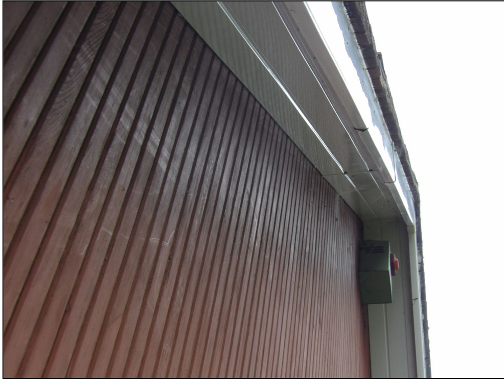
Figure 6. Example of gaps in the soffits/fascias on front elevation. 5 Greenside, Crowthorne. 17.03.26
