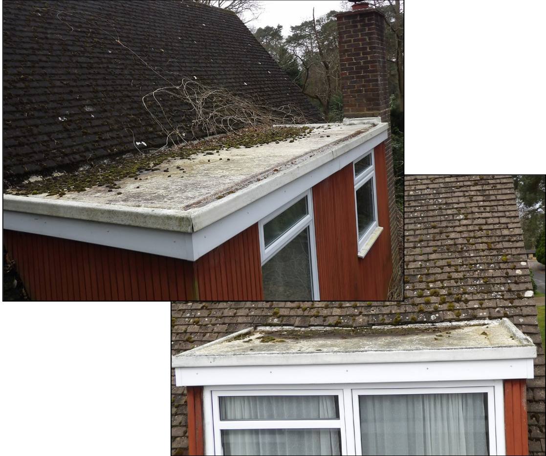
Figure 8. Example moulded plastic covering of dormer windows. 5 Greenside, Crowthorne. 17.03.26
