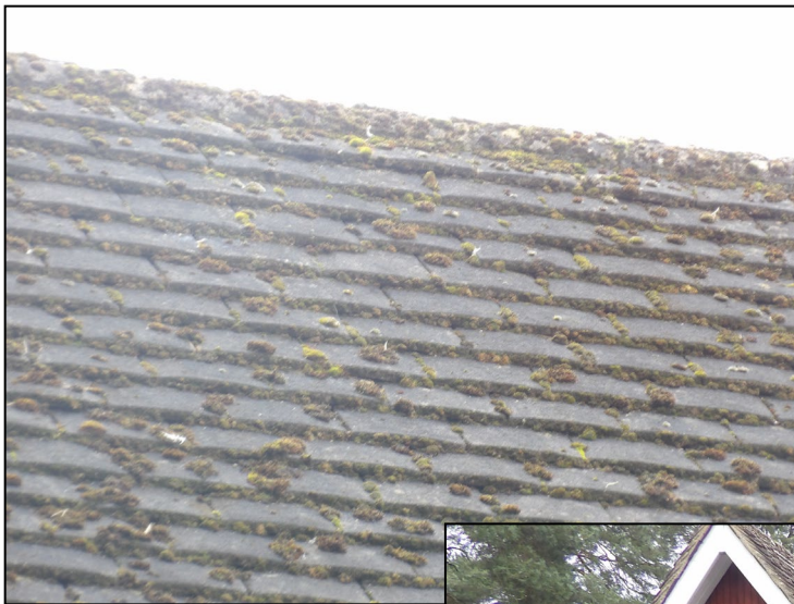
Figure 5. Example sealed ridge tiles and verges. 5 Greenside, Crowthorne. 17.03.26
