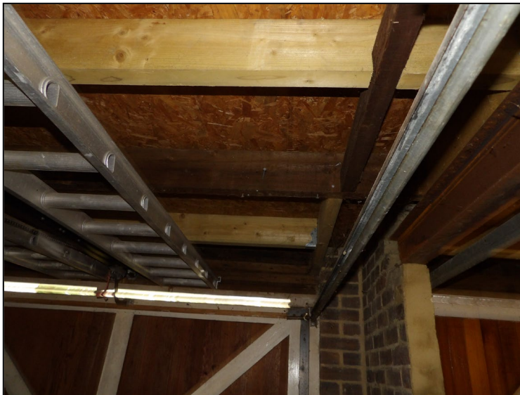
Figure 14. Example boarded ceiling of garage and storeroom. 5 Greenside, Crowthorne. 17.03.26
