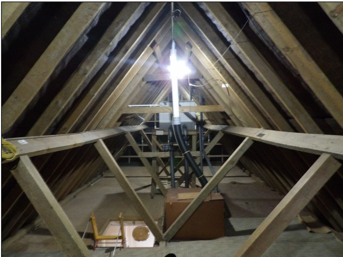
Figure 12. Example of loft space. 5 Greenside, Crowthorne. 17.03.26
