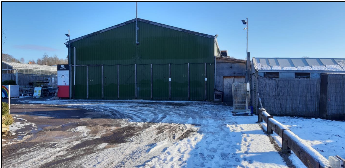
Fig. 4. Existing farm shop to be demolished (viewed from the existing car park), with existing glasshouse to be demolished on either side.
