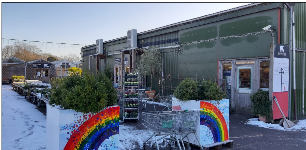
Fig. 3. Existing farm shop to be demolished.
