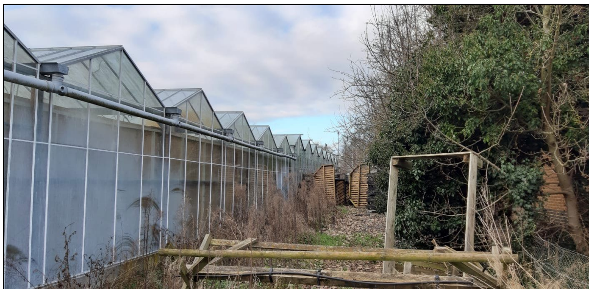
Fig. 2. Existing glasshouses to be demolished.
