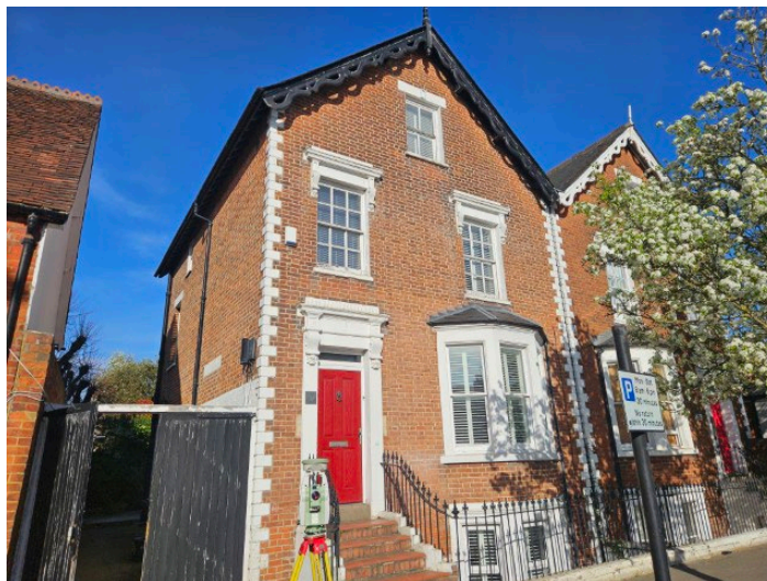
Photo 1 – View of front/side elevation (southwest)
