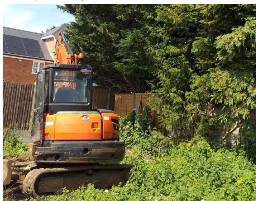
During the site visit an excavator was used to carry out three trial pits along the south western boundary of the site, beyond which lay the old engineering works. The locations are shown
