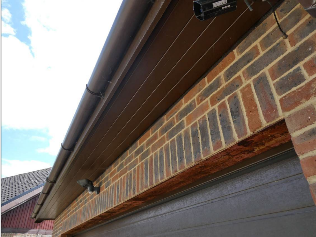
Figure 13. Soffits and fascias on garage. West Greylake, Part Lane, Riseley. 06.05.24
