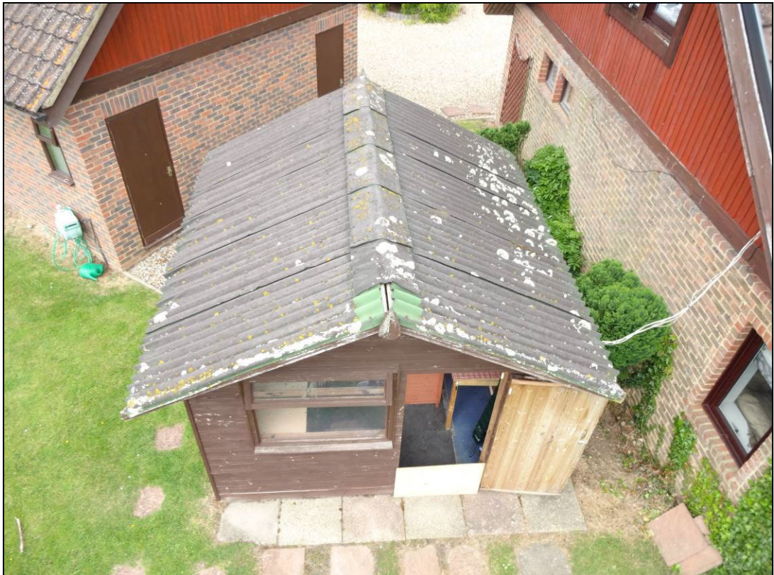
Figure 16. Roof of shed. West Greylake, Part Lane, Riseley. 06.05.24
