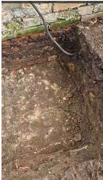
Photo 4a: Main House Foundation Trial Pit
