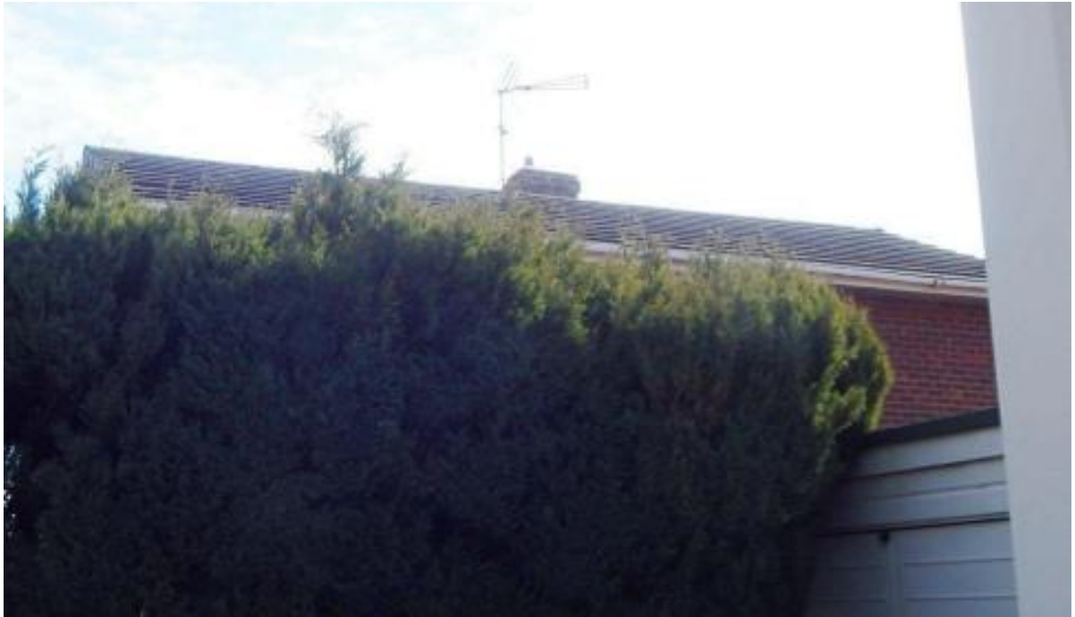
Image 5 – North facing elevation of the property
