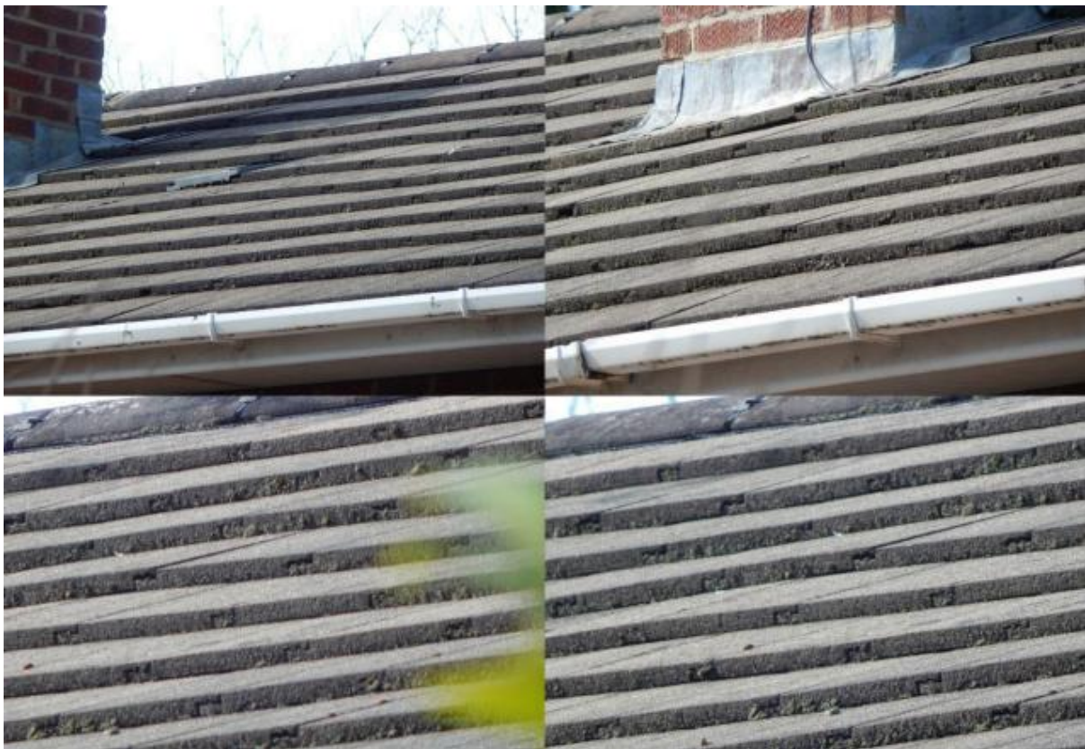
Image 4 – Close view of the South facing roof coverings
