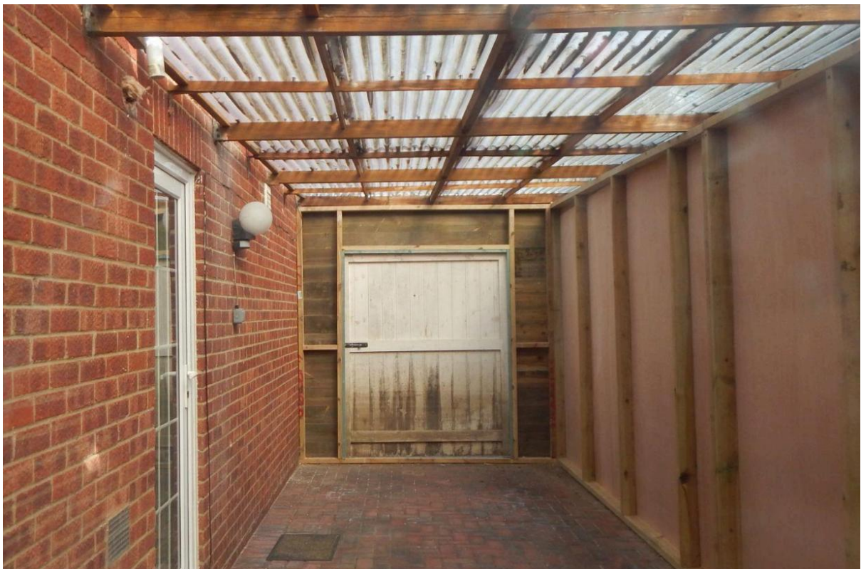
Image 8 – Internal view from below the fabricated roof covering section of the property
