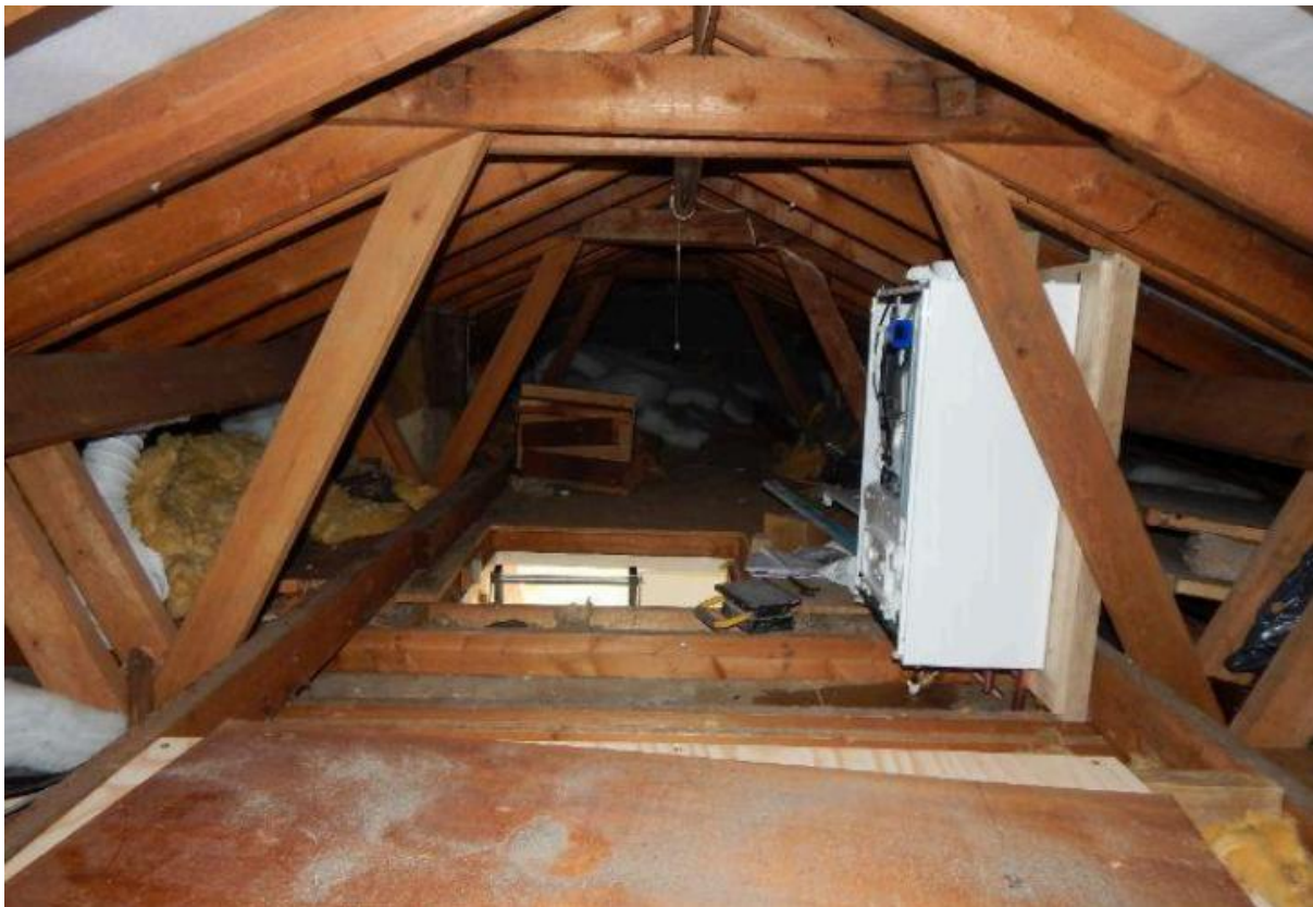
Image 9 – Internal view from within the main upper roof void spaces of the property
