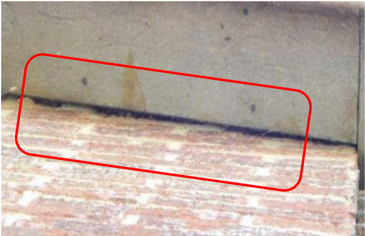
Image 7 – Further views of the eaves coverings which look to provide access opportunities for bats within
