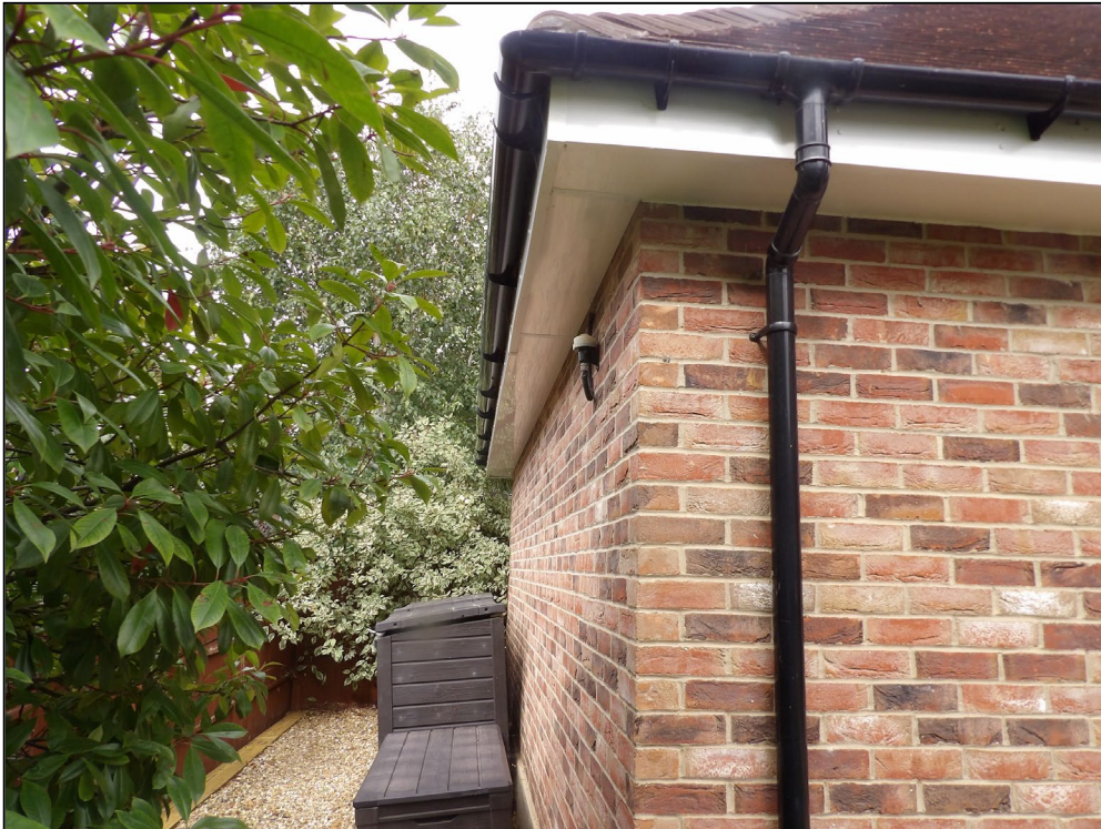
Figure 12. Example sealed uPVC soffits and fascias on garage. 4 Dearlove Place, Shinfield. 30.07.25
