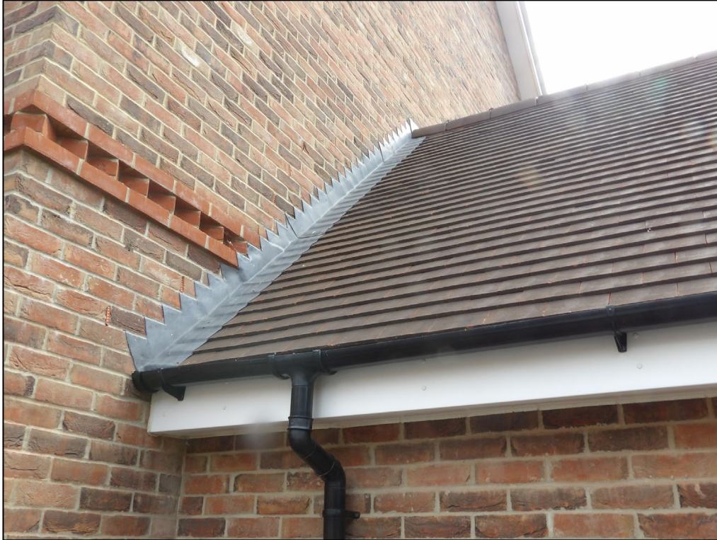
Figure 7. Example flush lead flashing. 4 Dearlove Place, Shinfield. 30.07.25
