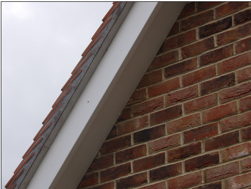
Figure 8. Example close fitted uPVC soffits and fascias. 4 Dearlove Place, Shinfield. 30.07.25
